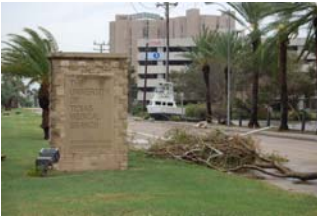
Front entrance at UT Medical Branch in Galveston, TX shows heavy damage. Photo from UTMB website
