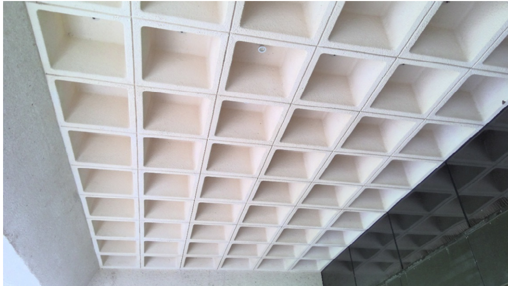
Photo 7: The shallower concrete waffle slab was also evident for the Third-Floor level at the exposed exterior corridor all around the perimeter of the entire building.
