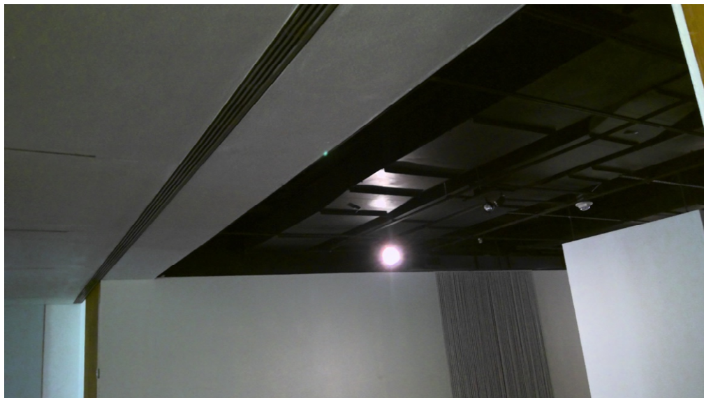
Photo 14: For the First-Floor supported by the Second-Floor framing, a cloud ceiling was observed with a suspended channel system without the lay-in fiberboard at the main corridor.
