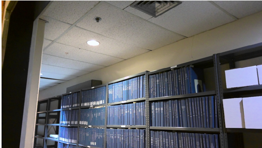
Photo 21: For the Third-Floor supported by the concrete Low Roof framing, lay-in ceiling was observed for typical office spaces, lounges, conferences rooms and miscellaneous rooms for workspaces and light storage rooms.
