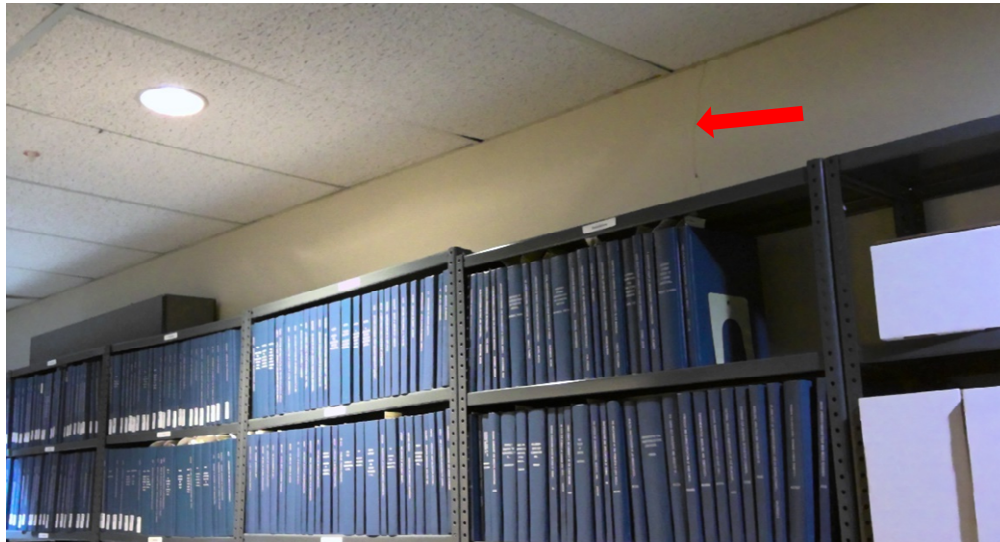
Photo 30: At the request of the Facilities Project Coordinator, cracking was observed within the gyp-board wall within the large storage room. This cracking was due to the gyp-board passing over the expansion joint without a metal expansion joint cover within the gyp-board wall.
