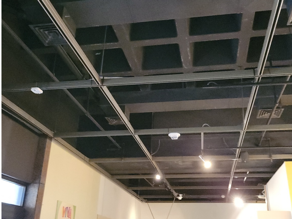
Photo 17: For the exhibit Second-Floor supported by the Third-Floor framing, a cloud ceiling was observed with a suspended channel system without the lay-in fiberboard throughout the entire floor within the interior of the building.
