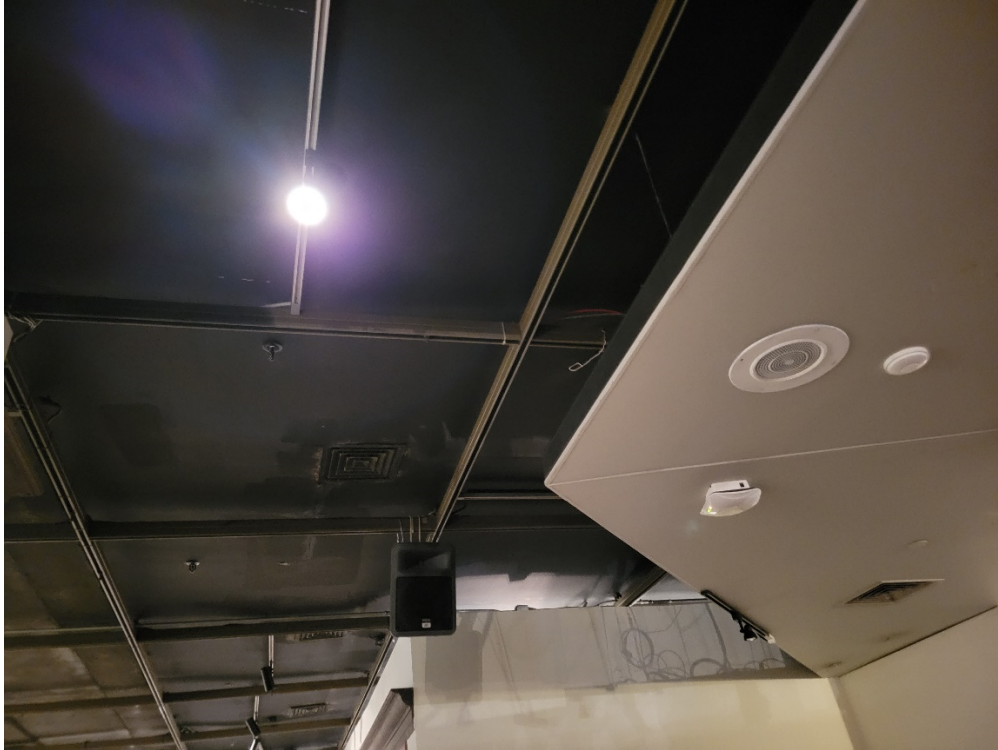
Photo 19: For the exhibit Second-Floor supported by the Third-Floor framing, a double gyp-board ceiling was observed with a second layer of gyp-board supported by the upper layer of gyp-board within an irregular transition layout around the dome opening.
