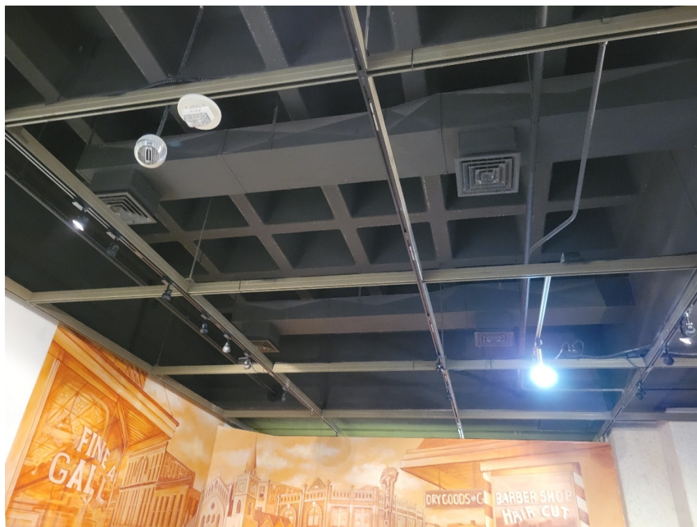
Photo 6: The deeper concrete waffle slab was evident for the Third-Floor framing from below throughout the exhibit Second-Floor level through the open cloud ceiling.
