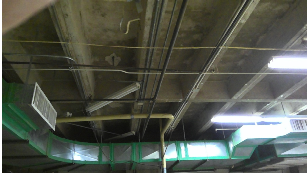
Photo 5: A concrete one-way joist system was evident for the support of the exhibit Second-Floor level.
