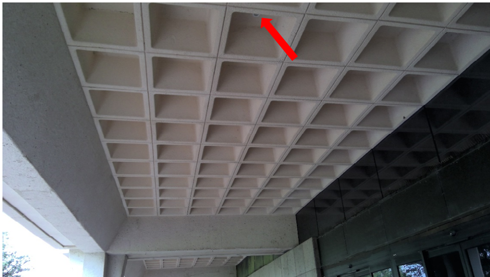
Photo 20: For the exterior corridor at the exhibit Second-Floor supported by the Third-Floor framing, minimal lighting but no other collateral load was observed for the exposed exterior shallow waffle slab concrete framing.
