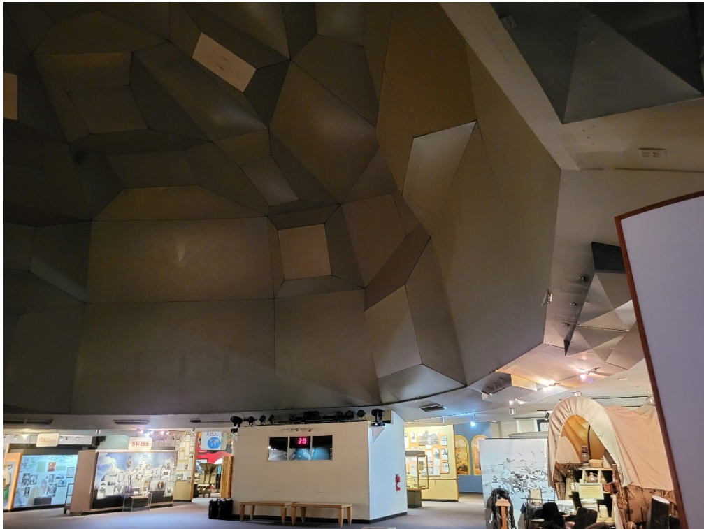
Photo 10: The dome ceiling was evident looking up from the exhibit Second-Floor level extending through the opening on the Third-Floor level, the opening on the concrete Low Roof level, and on up to the underside of the steel High Roof level.
