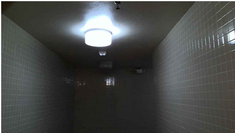
Photo 12: For the First-Floor supported by the Second-Floor framing, gyp-board ceiling was observed for all restrooms, open areas near the entries into the First-Floor level, small storage rooms, and miscellaneous rooms that were too small to install a lay-in ceiling.
