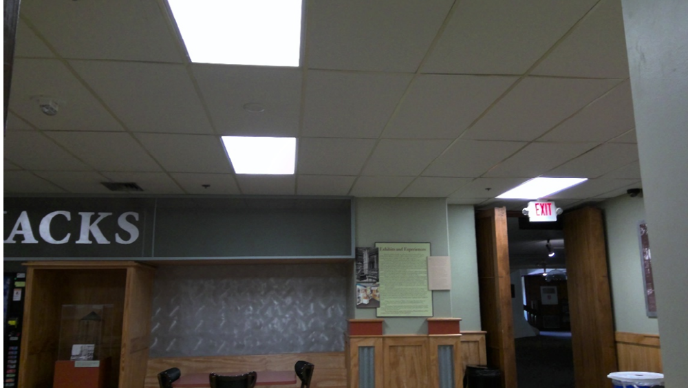
Photo 11: For the first floor supported by the Second-Floor framing, lay-in ceiling was observed for typical office spaces, lounges, conferences rooms and miscellaneous rooms for workspaces and light storage rooms.
