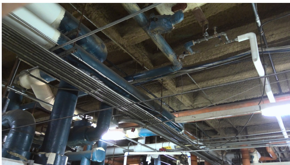
Photo 16: For the First-Floor, there were exposed areas of the Second-Floor framing observed with limited spray-on insulation in random mechanical rooms.
