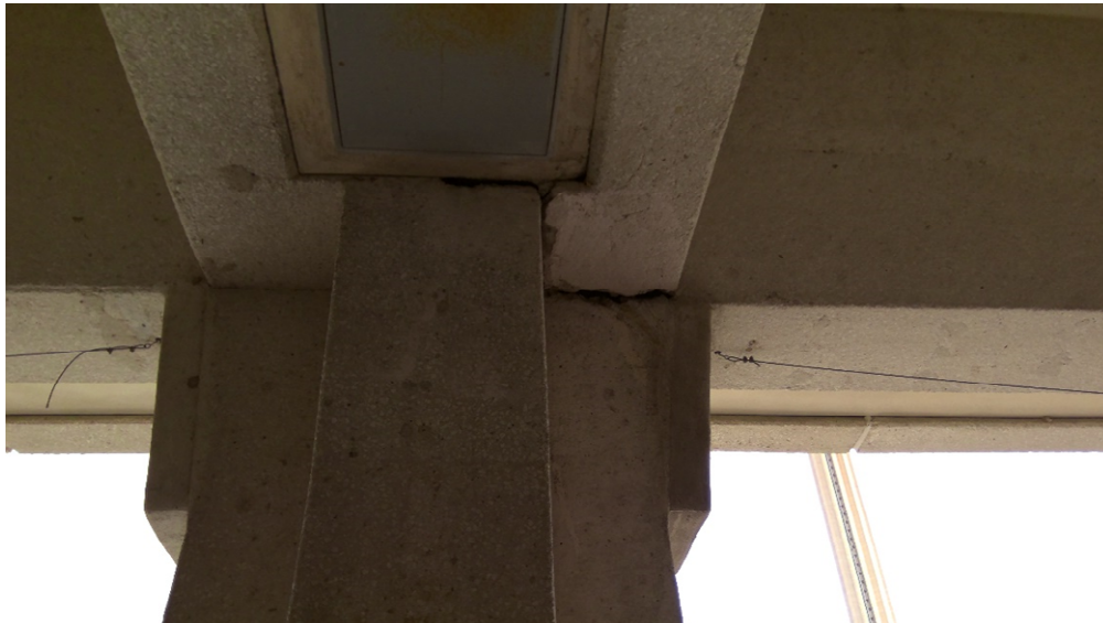
Photo 32: An existing structural repair was observed due to spalling of the concrete at an exterior concrete column at an expansion joint utilizing a corbel type condition at the top of the concrete column located on the West side of the building at the expansion joint furthest South on the exhibit Second-Floor level exterior corridor.
