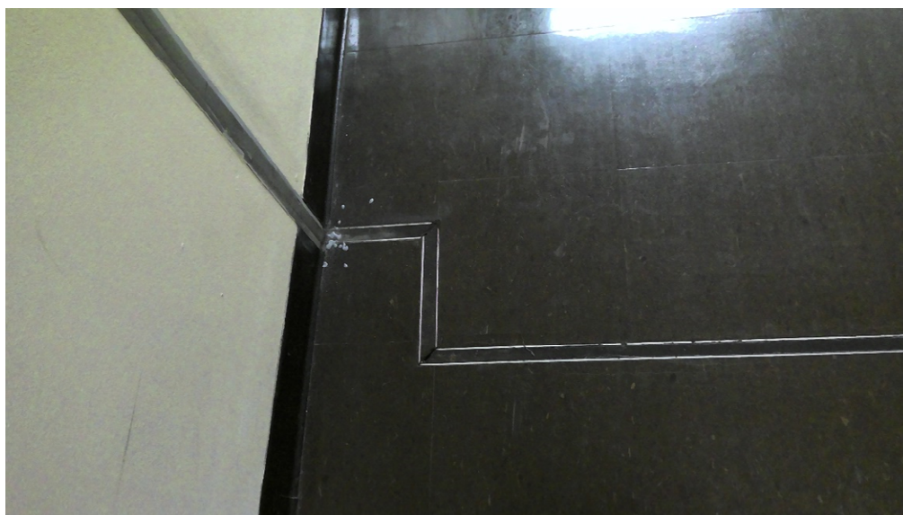
Photo 26: For the Second-Floor, the expansion joint was observed from above on the Third-Floor which extends from the Second-Floor and the upper gyp-board walls which follows the details provided within the existing structural drawings.
