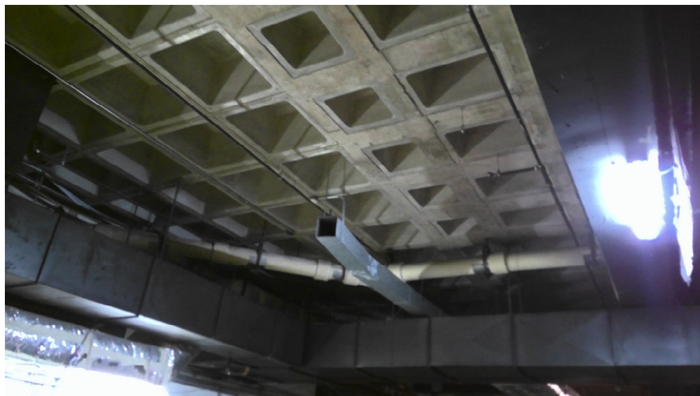
Photo 8: A concrete waffle slab was evident for the low concrete roof level along with the widened joists along the perimeter of the dome opening for support of the steel High Roof above.
