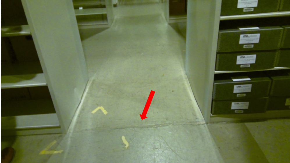
Photo 23: A 3" floor depression was designated on the existing structural drawings which marks the transition of the shallow and deeper joists along the entire perimeter of the building which appeared to have a 3" concrete topping over the exterior corridor below.
