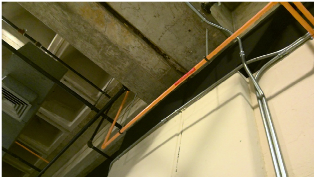
Photo 28: For the concrete Low Roof framing, the double concrete beams were observed, one on each side of the expansion joint, which follow the details provided within the existing structural drawings.
