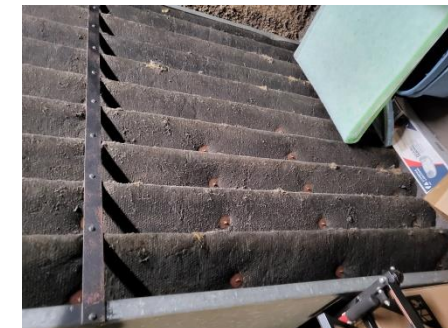
12. AH 1, Not properly maintained
