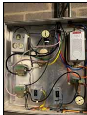
PHOTOGRAPH 112 – AHU 10 DDC for pneumatic system
