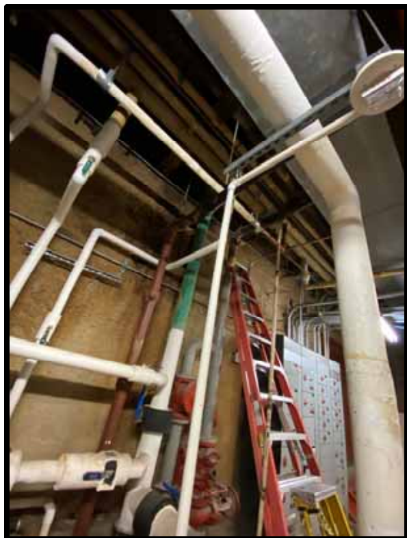
PHOTOGRAPH 281 – Typical domestic cold and hot water piping.
