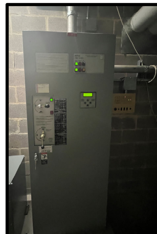
PHOTOGRAPH 212 – Bypass Isolation Transfer Switch
