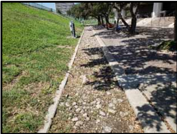
PHOTOGRAPH 33 – View of probable French drain at the base of the berm.
