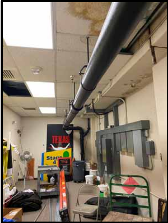
PHOTOGRAPH 243 – Typical cast iron piping. Possible leak from sprinkler pipe.
