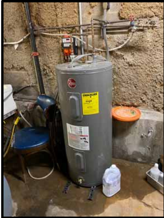
PHOTOGRAPH 302 – Mechanical room water heater. CW line needs heat trap, vacuum breaker, and expansion tank. Water heater needs to be in a drain pan on housekeeping pad.
