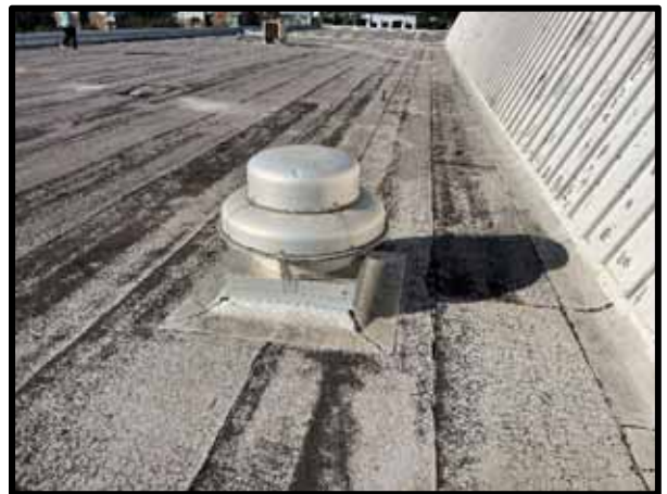
PHOTOGRAPH 60 – View of the granule loss taking place in the modified bitumen roofing membrane.
