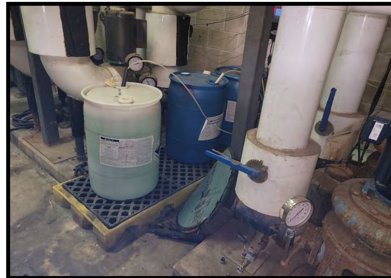
Photo 12. Water treatment chemicals for cooling tower.
