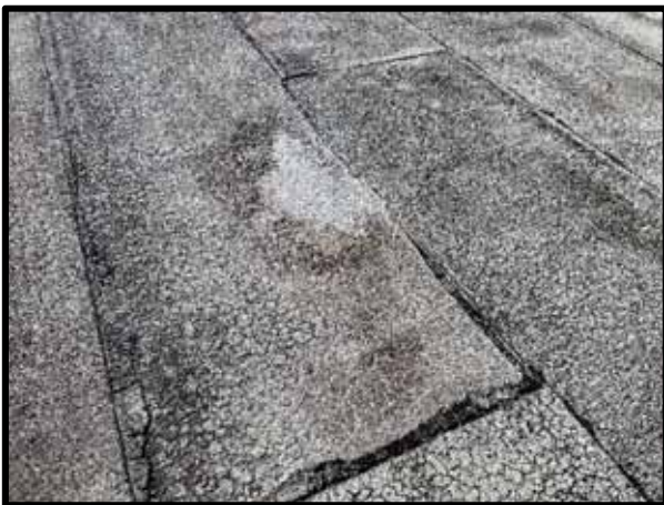
PHOTOGRAPH 59 – View of alligatoring and membrane shrinkage in the modified bitumen roof membrane.
