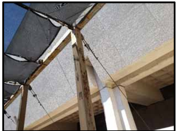
PHOTOGRAPH 36 – View of structural steel framing of the canopy structure. There is visible oxidation and possible corrosion of the steel.
