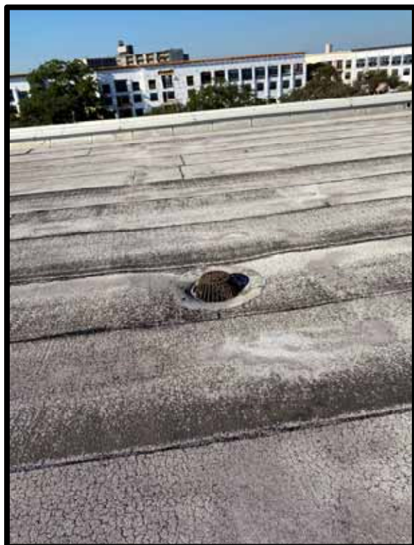
PHOTOGRAPH 270 – Typical roof drain scupper.
