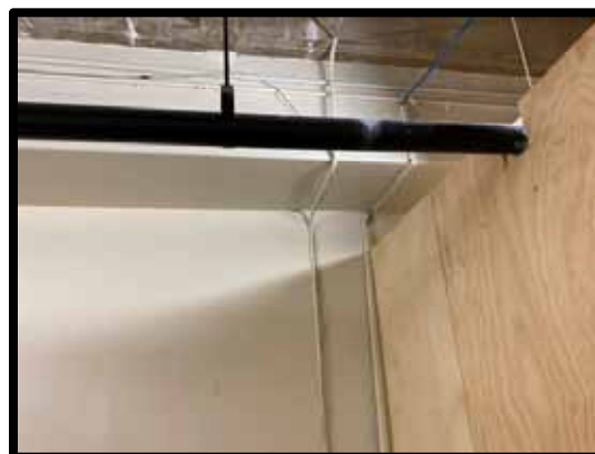
PHOTOGRAPH 238 – Typical cast iron piping.
