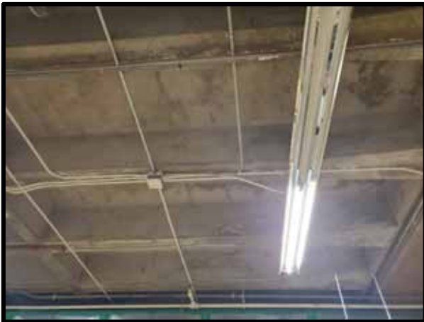
PHOTOGRAPH 51 – View of second floor framing with staining that may indicate moisture infiltration.
