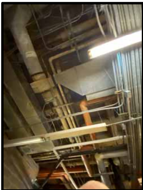
PHOTOGRAPH 289 – Typical domestic cold and hot water piping.
