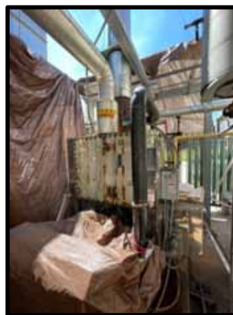
PHOTOGRAPH 102 - Corrosion on Boiler 1
