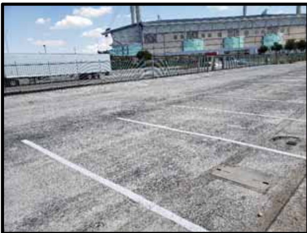
PHOTOGRAPH 5 – General view of parking lot on the east side of the property. Pavement is in fair condition with evidence of full-depth patch repairs, transverse and longitudinal cracking, raveling, and rutting.
