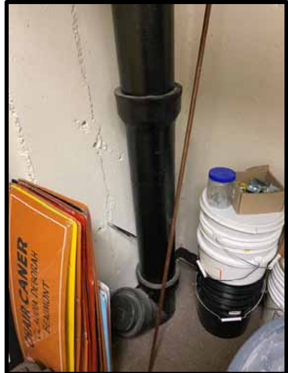
PHOTOGRAPH 245 – Typical cast iron piping.
