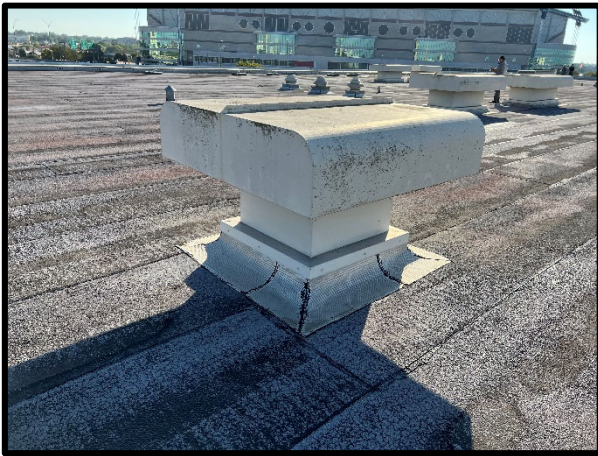
PHOTOGRAPH 61 – Overview photo of typical roof penetration with aluminum clad base flashing. Also noted in photo is the presence of granule loss and membrane alligatoring in the modified bitumen roof membrane.
