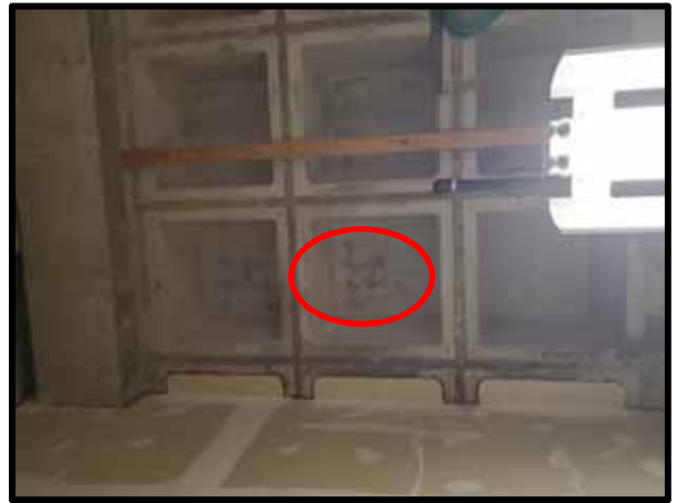
PHOTOGRAPH 50 - View of roof framing with possible moisture staining.
