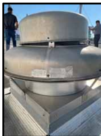
PHOTOGRAPH 176 - EF-12 Top Cap missing hardware
