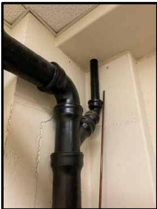
PHOTOGRAPH 244 – Typical cast iron piping.
