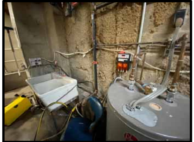
PHOTOGRAPH 304 – Water heater, utility sink, and associated piping.
