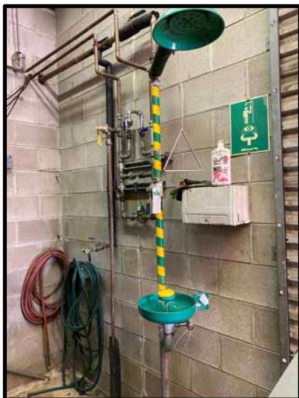
PHOTOGRAPH 293 – Central plant emergency eyewash station.
