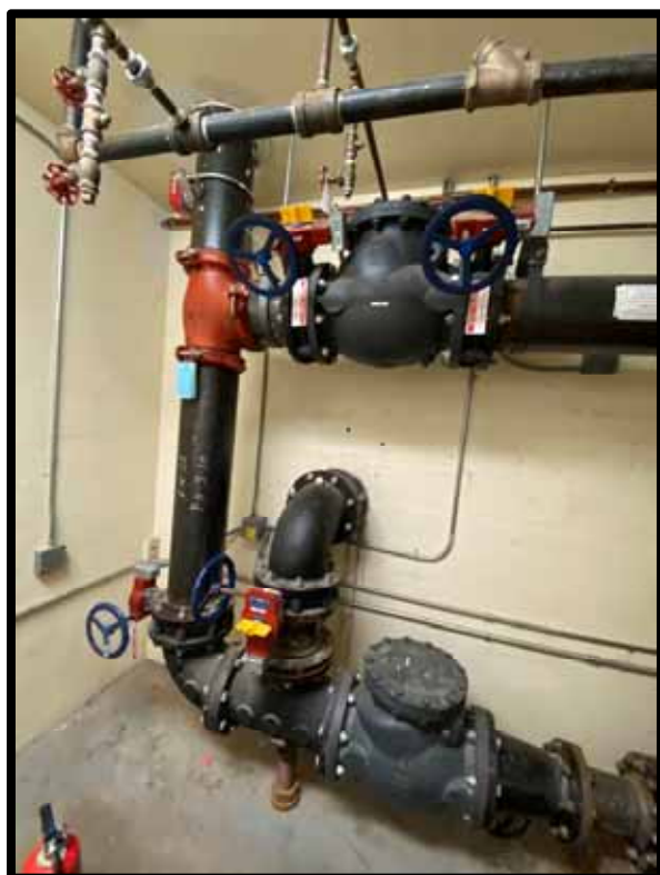
PHOTOGRAPH 322 - Fire pump piping.
