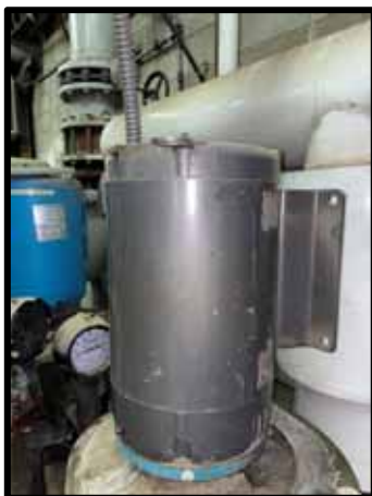
PHOTOGRAPH 99 – Chill Water Pump 1 Motor
