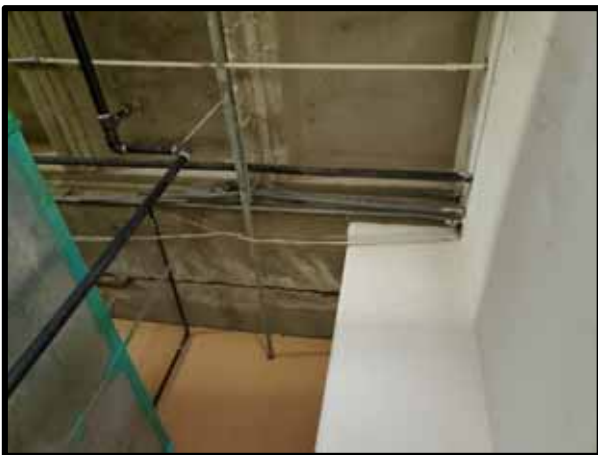
PHOTOGRAPH 53 – View of expansion joint through the first floor framing with possible moisture staining and efflorescence.
