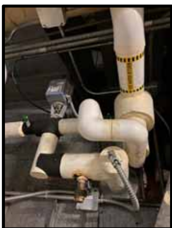
PHOTOGRAPH 135 – AHU 4 HW Supply with electronic actuator
