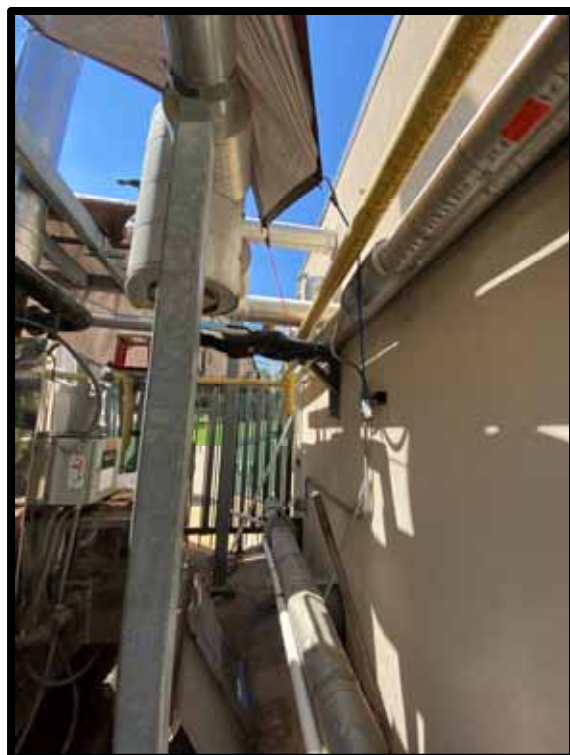
PHOTOGRAPH 312 – Natural gas manifold.
