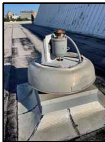
PHOTOGRAPH 174 - EF missing belt for belt-drive motor
