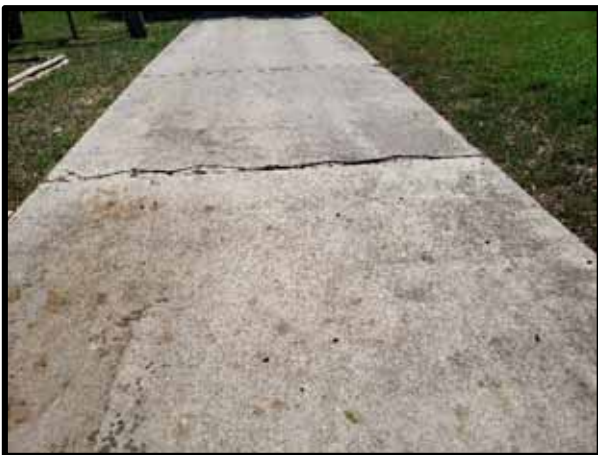
PHOTOGRAPH 11 – View of concrete sidewalk with a transverse crack the width of the sidewalk. There is spalled concrete between the crack and the joint.
