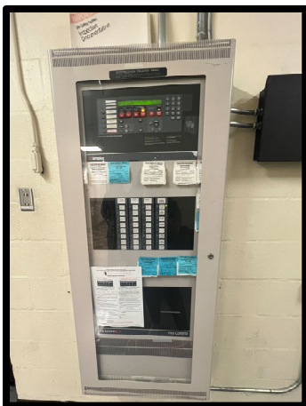
PHOTOGRAPH 211 – Fire Alarm Control Panel
