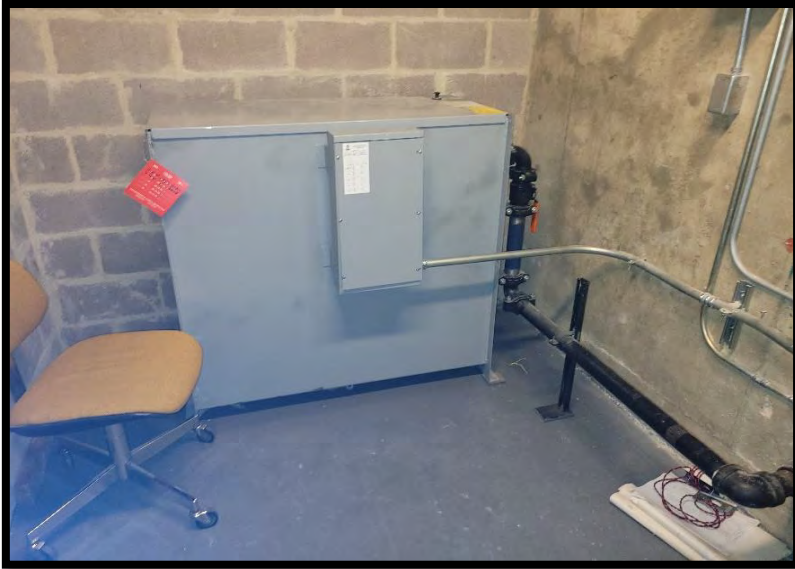
Photo 9. Elevator hydraulic reserve.
