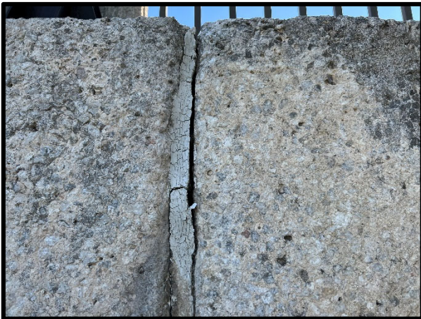
PHOTOGRAPH 69 – Sealant joint failure at the fountain and walkover bridge area.
