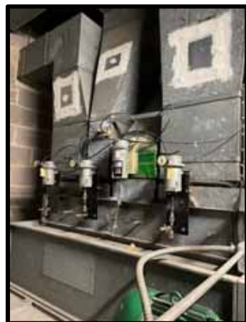
PHOTOGRAPH 118 – AHU 11 Pneumatic control system
