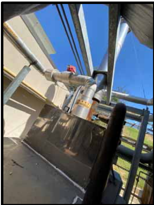
PHOTOGRAPH 307 – Boiler and natural gas piping.
