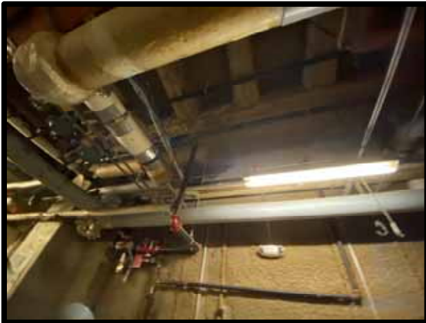
PHOTOGRAPH 285 - Typical domestic cold and hot water piping. Missing insulation.
