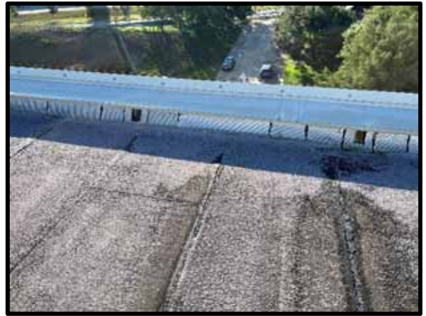
PHOTOGRAPH 56 – View of aluminum clad base flashing at the parapet wall conditions and the thru-wall scuppers used as the secondary/overflow drainage.
