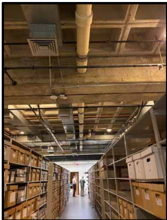
PHOTOGRAPH 273 – Typical roof drain piping.
