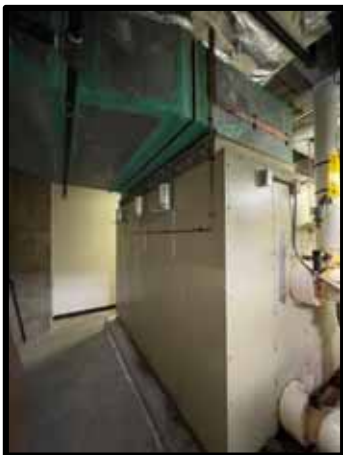
PHOTOGRAPH 121 – AHU 17 Pneumatically actuated damper system
