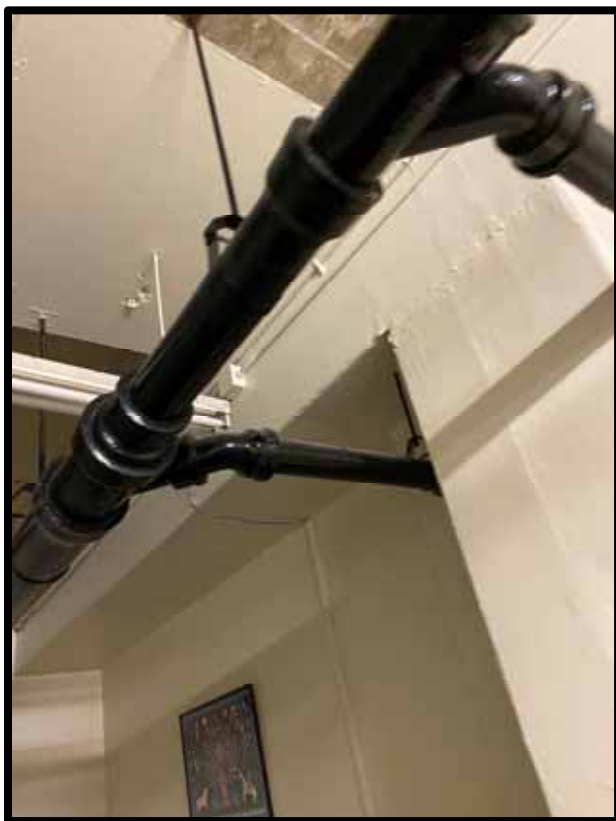
PHOTOGRAPH 240 – Typical cast iron piping.
