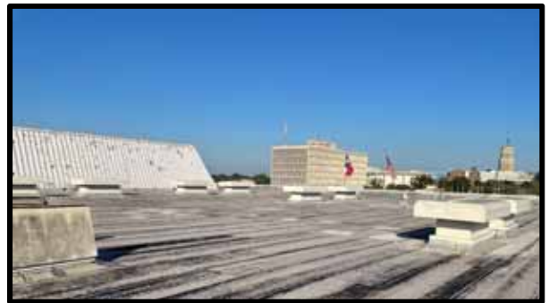
PHOTOGRAPH 170 - Array of outside air intake roof hoods on one side of the roof
