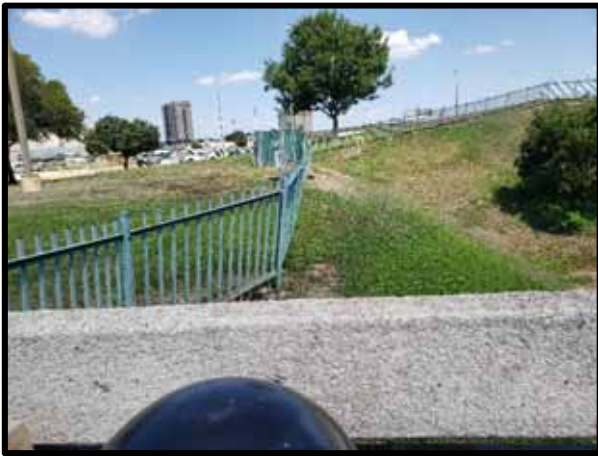
PHOTOGRAPH 31 – View of fencing at the northwest corner of the property. The fence is leaning and there is a section of fence that has been damaged.
