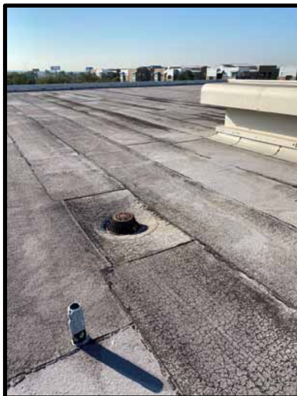
PHOTOGRAPH 271 – Typical roof drain scupper.
