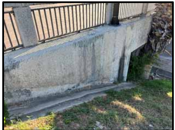
PHOTOGRAPH 341 – General view of retaining wall with moisture staining.
