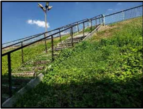
PHOTOGRAPH 25 – View of steps on the north side of the building that extend from the building. These steps are in poor condition and have been barricaded against pedestrian traffic.
