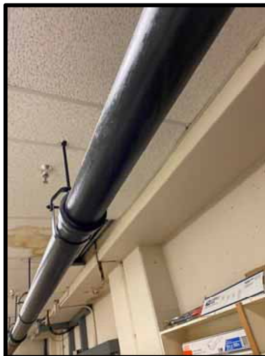
PHOTOGRAPH 242 - Typical cast iron piping.
