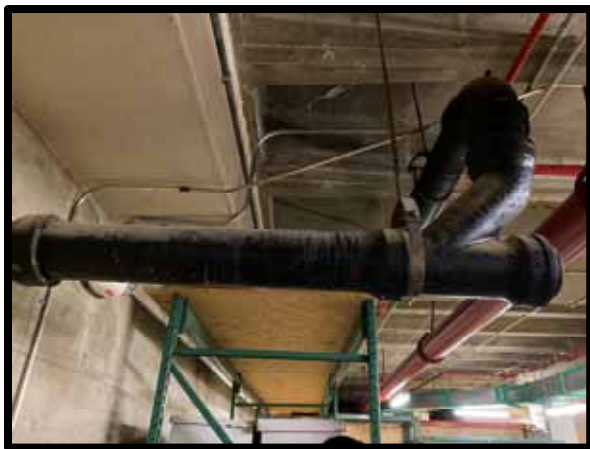
PHOTOGRAPH 233 – Typical cast iron piping.
