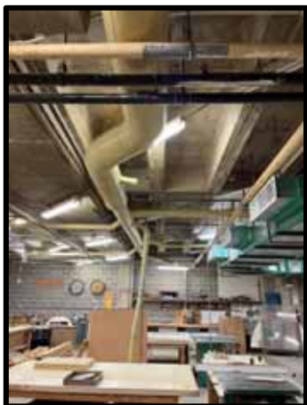
PHOTOGRAPH 185 – Dust collector system with drops at various workstations and machines
