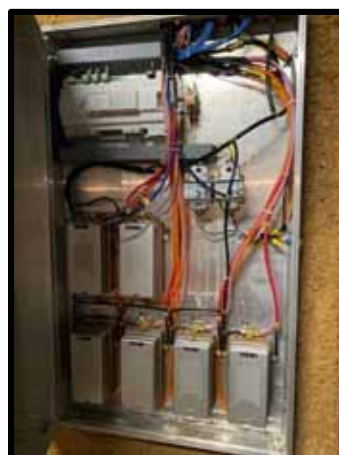
PHOTOGRAPH 134 - AHU 4 DDC to pneumatic controls system
