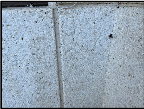
PHOTOGRAPH 67 – Wall panel joint condition at the pre-cast wall panels. Typical joint appears to be a masonry reveal joint that are in overall good condition.
