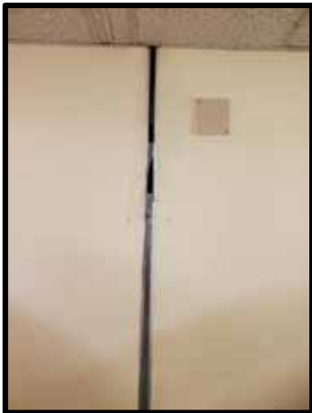
PHOTOGRAPH 45 – View of the expansion joint on the third floor in Corridor 3.04. There is distress in the joint sealant.
