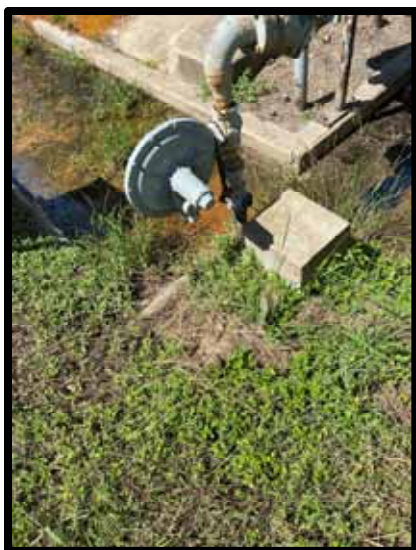
PHOTOGRAPH 310 – Gas regulator at central plant.
