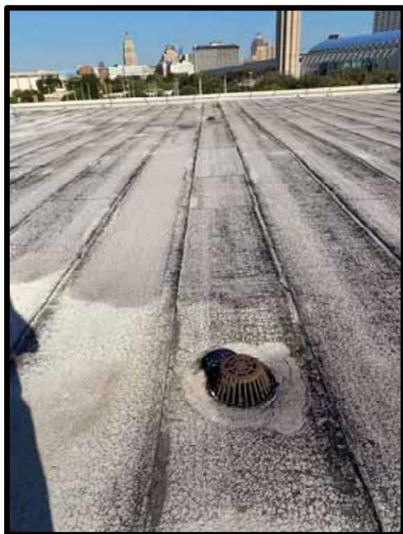
PHOTOGRAPH 278 – Typical roof drain scupper.
