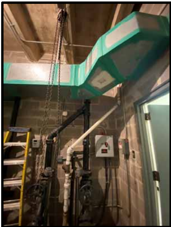
PHOTOGRAPH 255 – Sump pump piping.
