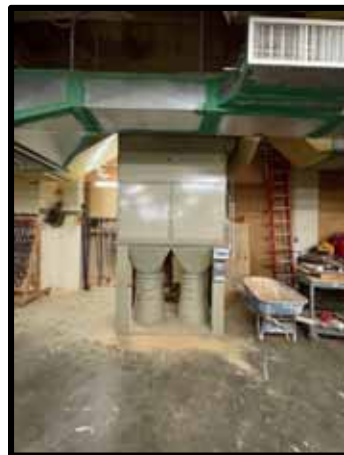
PHOTOGRAPH 182 - Dust collector Unit
