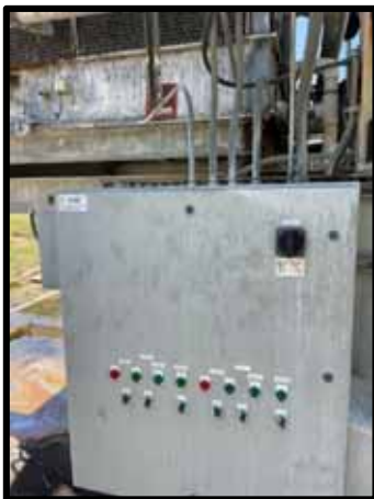
PHOTOGRAPH 109 – Cooling Tower Control Panel
