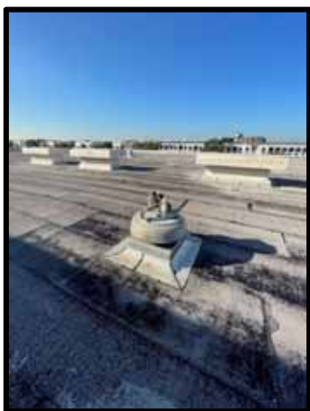
PHOTOGRAPH 173 – Non-operational ventilator with removed top cap
