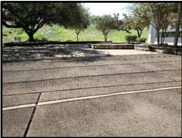
PHOTOGRAPH 15 – View of concrete patio with cracks in the concrete. There is no joint sealant between concrete panels.
