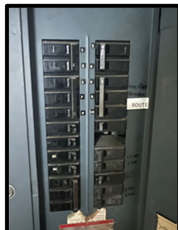
PHOTOGRAPH 194 – Example of Panel missing blank cover
