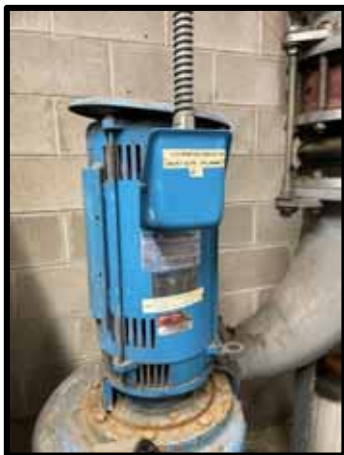
PHOTOGRAPH 91 – Condenser Pump 2 wear due to service life
