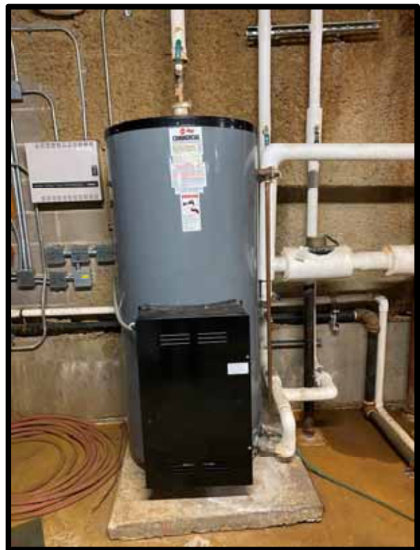
PHOTOGRAPH 305 – Commercial water heater for building hot water supply.
