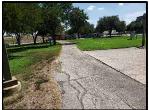
PHOTOGRAPH 18 – View of asphalt sidewalk that extends along the east side of the property. Pavement is in poor condition with transverse and longitudinal cracks and edge raveling.
