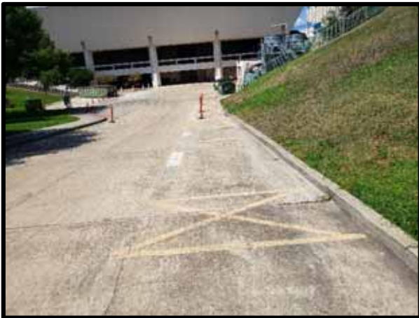
PHOTOGRAPH 9 – View of the service drive with transverse and longitudinal cracks. Joint sealant is in poor condition.
