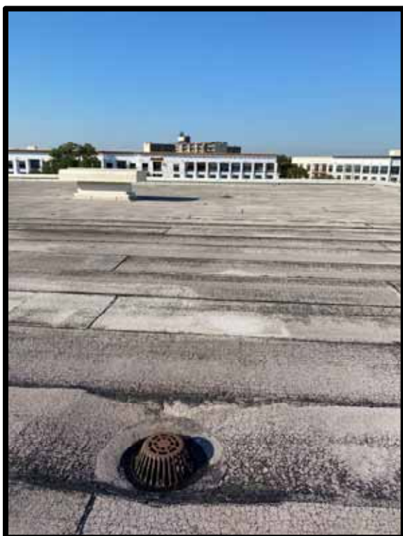
PHOTOGRAPH 268 – Typical roof drain scupper.
