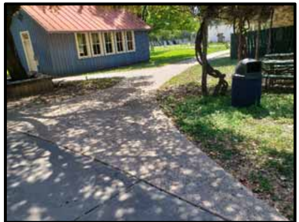
PHOTOGRAPH 12 – General view of the concrete sidewalk. There is exposed aggregate. Joint sealant is not present.
