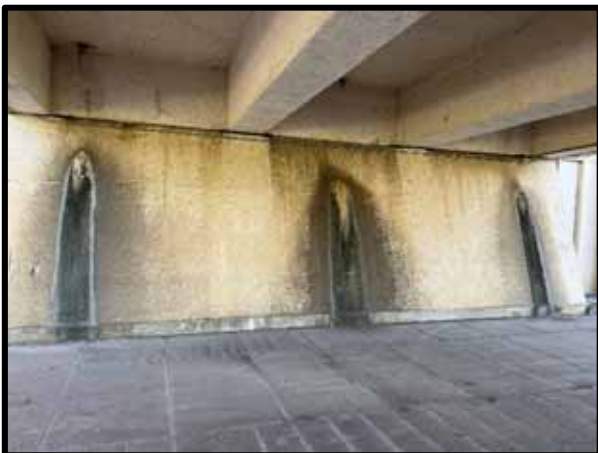
PHOTOGRAPH 340 – View of moisture staining on retaining wall at pipe penetrations.
