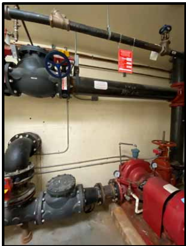
PHOTOGRAPH 321 – Fire pump piping.
