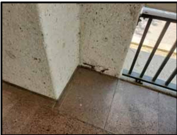
PHOTOGRAPH 47 – Example of concrete spall with exposed rebar.
