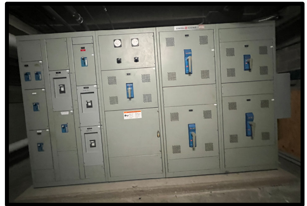
PHOTOGRAPH 190 – Main Switchboard and Distribution Section
