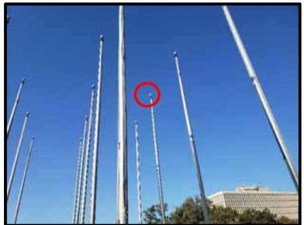
PHOTOGRAPH 42 – Example of flagpole with bent top.
