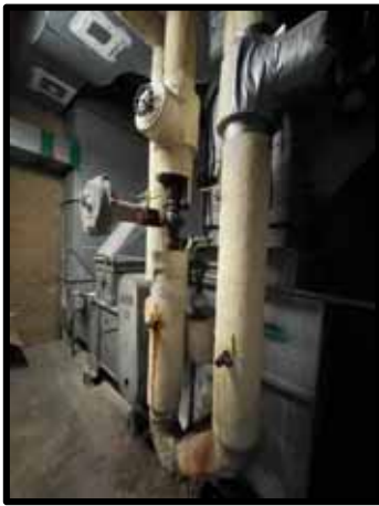
PHOTOGRAPH 119 – AHU 11 Deteriorated piping and insulation, incomplete insulation
