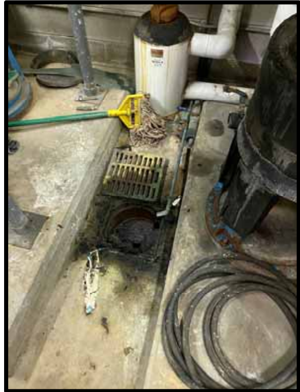
PHOTOGRAPH 266 – Central plant floor sink. Recommend replacement.
