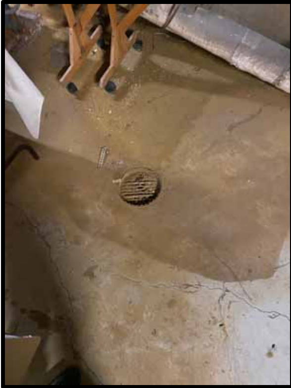
PHOTOGRAPH 263 - Mechanical room floor drain. Recommend replacement.
