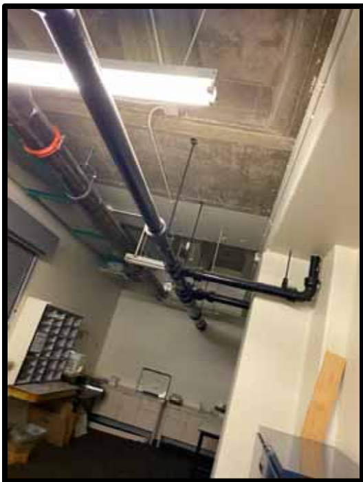
PHOTOGRAPH 239 – Typical cast iron piping.
