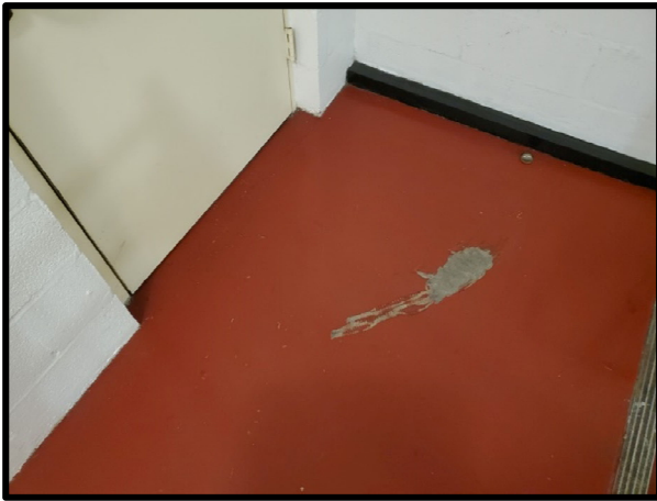
PHOTOGRAPH 73 – Example of distress to the concrete-floor staining. This type of distress is typical for buildings of this age and was only observed at isolated locations.
