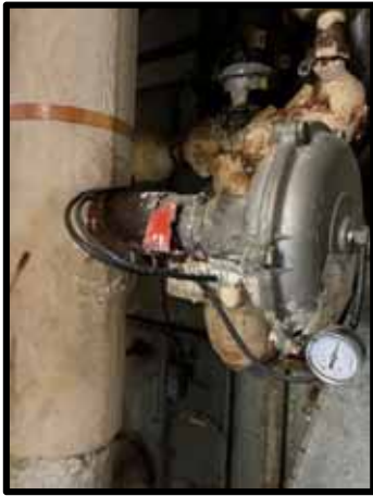
PHOTOGRAPH 113 – AHU 10 Corrosion on hydronic piping and instrumentation
