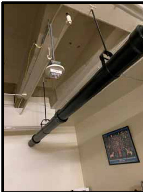
PHOTOGRAPH 241 - Typical cast iron piping and Simplex 4100U Fire Alarm System
