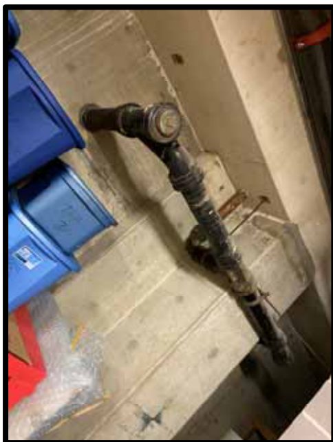
PHOTOGRAPH 252 – Typical cast iron piping.
