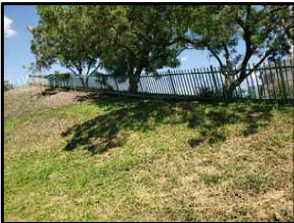
PHOTOGRAPH 29 – View of fence on the top of the berm adjacent to the service drive. Fence is leaning and several of the footings appear to be undermined.
