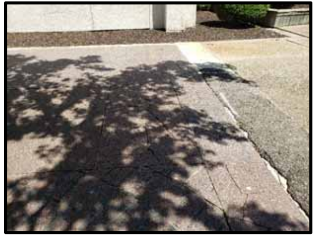
PHOTOGRAPH 20 – View of granite sidewalk with cracks in the granite slabs.
