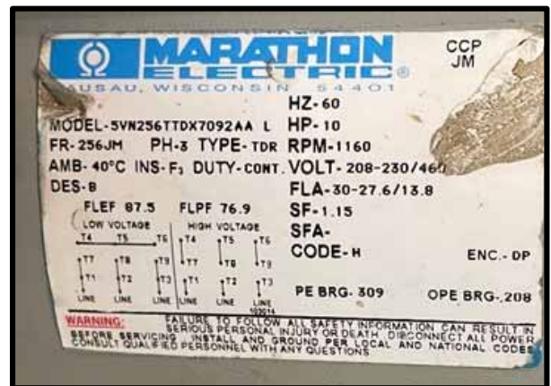
PHOTOGRAPH 90 - Condenser Pump 1 Motor Tag
