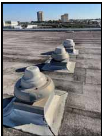
PHOTOGRAPH 171 – Operational rooftop ventilators
