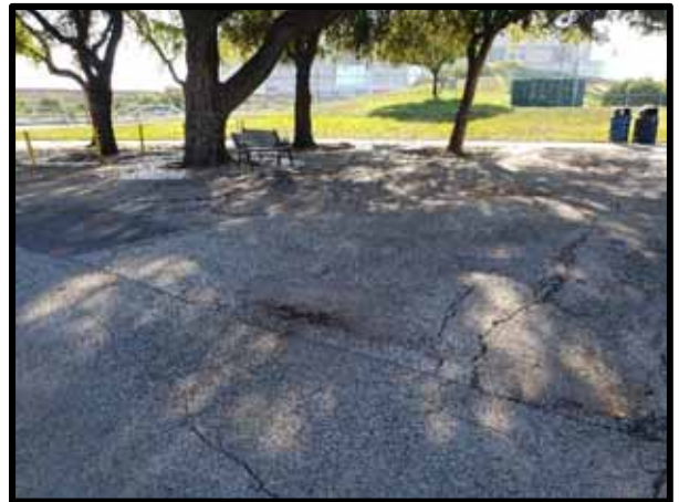
PHOTOGRAPH 16 – General view of asphalt-paved seating area on the west side of the property. Asphalt paving is in poor condition.
