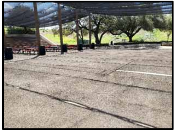
PHOTOGRAPH 14 – General view of the patio area on the south side of the building. There is not joint sealant between concrete panels.
