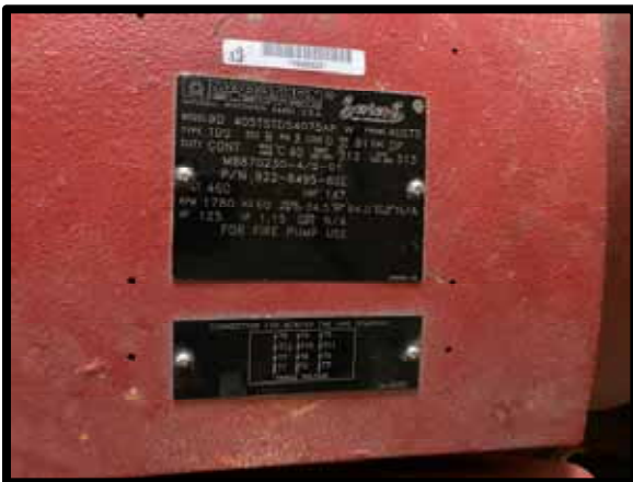
PHOTOGRAPH 315 – Fire pump nameplate.
