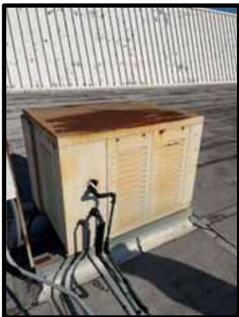
PHOTOGRAPH 181 – Piping insulation to unit showing extreme wear
