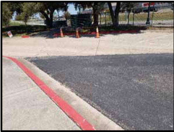
PHOTOGRAPH 7 – General view of the entrance to the service drive on the south side of the property. Concrete pavement is in fair condition with corner cracks and transverse cracks.
