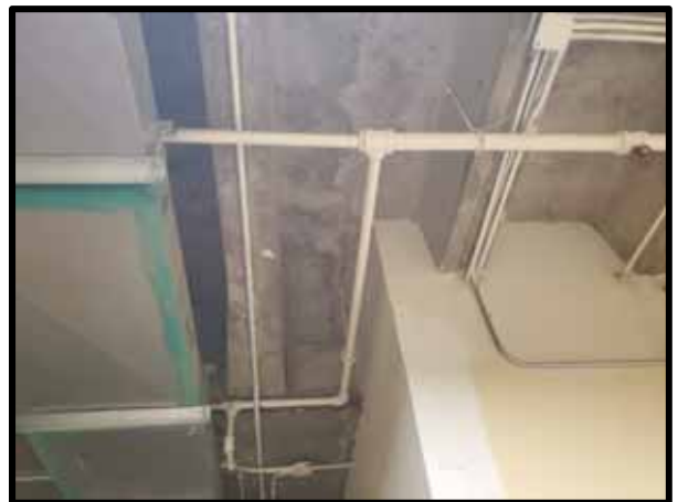
PHOTOGRAPH 54 – View of second floor framing with staining that may indicate moisture infiltration.
