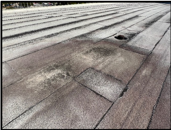
PHOTOGRAPH 63 – Ponding condition observed at the roof drains at the projection room roof area (Typical).
