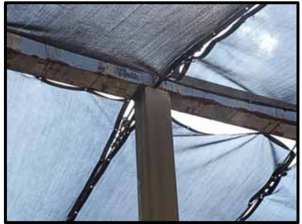
PHOTOGRAPH 38 - View of structural steel framing of the canopy structure. There is visible oxidation and possible corrosion of the steel.
