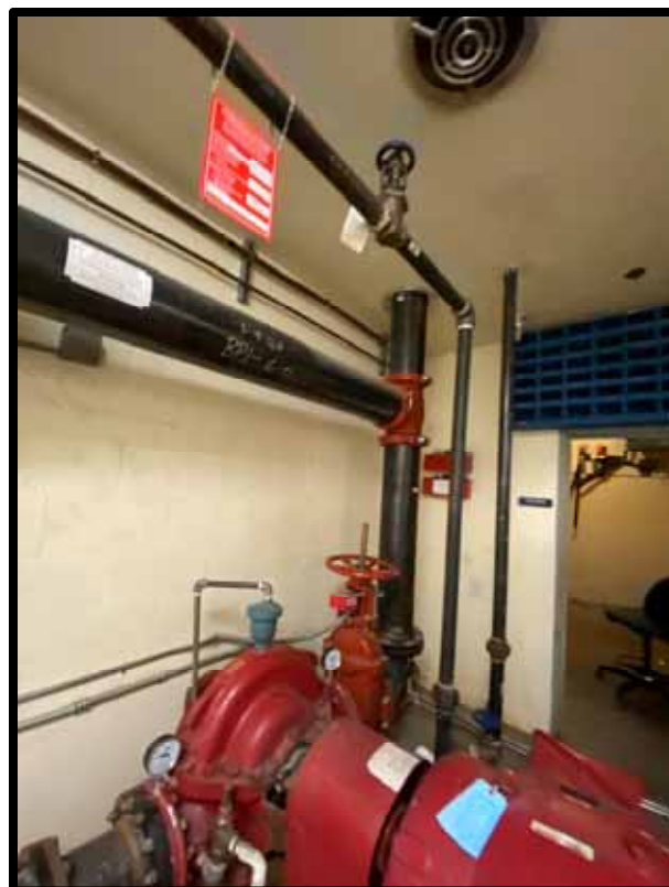
PHOTOGRAPH 323 - Fire pump piping.
