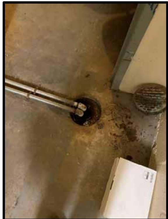
PHOTOGRAPH 316 – Fire pump condensate drain.
