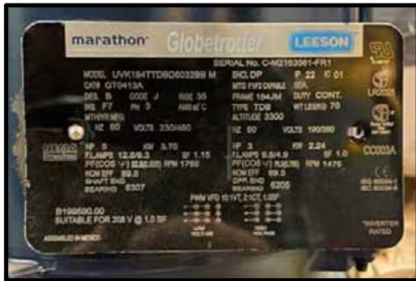
PHOTOGRAPH 95 – Hot Water Pump 1 Motor Tag
