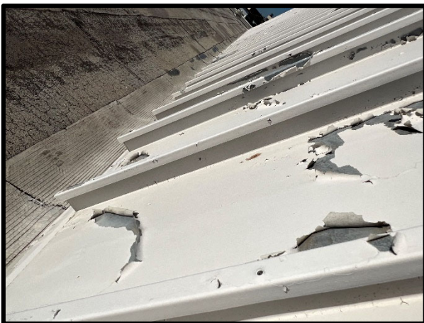
PHOTOGRAPH 65 – Where the metal wall panels are installed at the projection room, the exterior paint that appears to be installed over the galvanized metal panels is beginning to peel and flake away from the metal panels.
