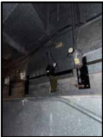
PHOTOGRAPH 127 – AHU 6 Pneumatic Dampers
