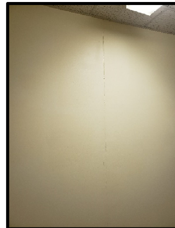
PHOTOGRAPH 78 – Example of vertical crack in Corridor 3.04.C4. This type of distress is typical for buildings of this age and was only observed at isolated locations.
