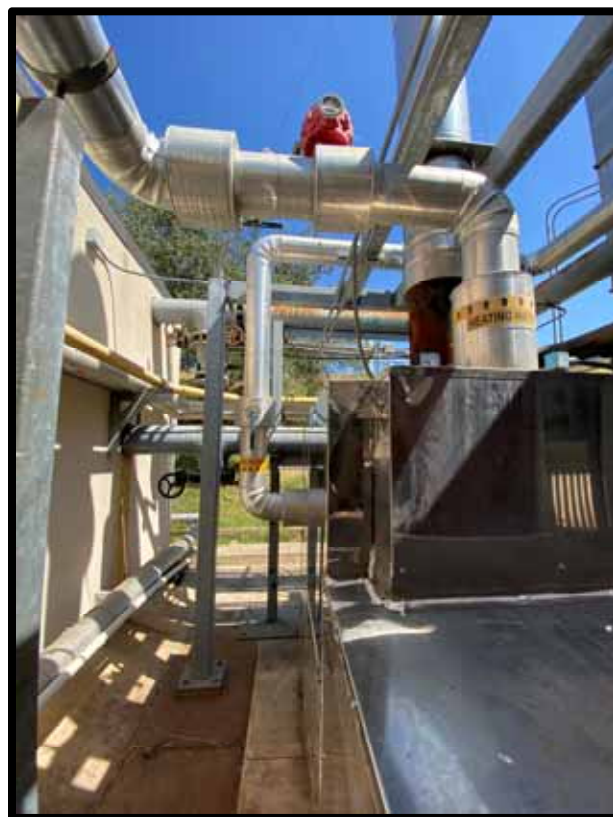
PHOTOGRAPH 313 – Boiler and natural gas piping.
