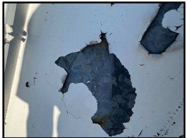
PHOTOGRAPH 66 – Where the metal wall panels are installed at the projection room, the exterior paint that appears to be installed over the galvanized metal panels is beginning to peel and flake away from the metal panels.
