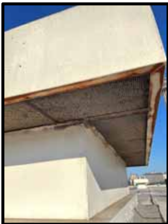
PHOTOGRAPH 169 – Buildup of particulates on grills of outside air intake roof hood
