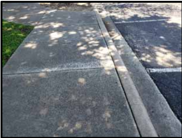
PHOTOGRAPH 27 – Example of concrete curb with isolated cracks.
