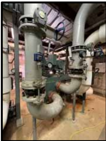
PHOTOGRAPH 85 – Piping and instrumentation to Chiller 1
