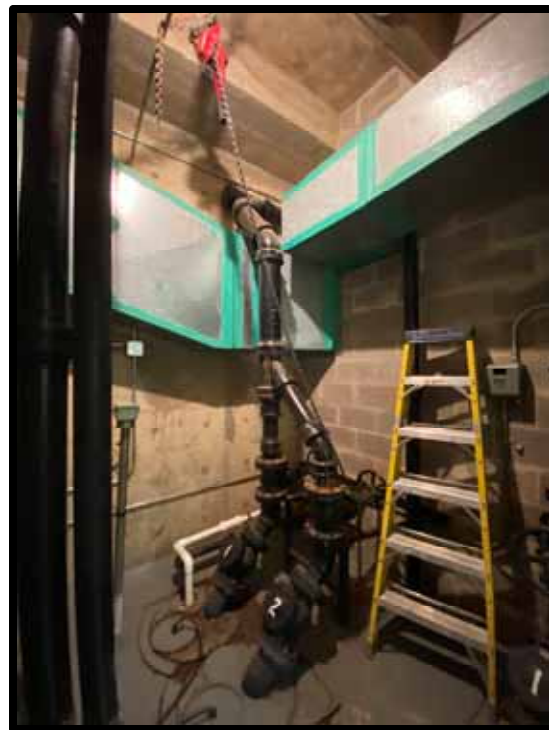
PHOTOGRAPH 257 - Sump pump piping.
