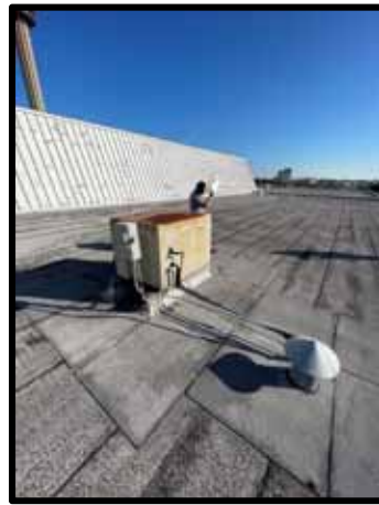
PHOTOGRAPH 180 - Decommissioned condenser unit
