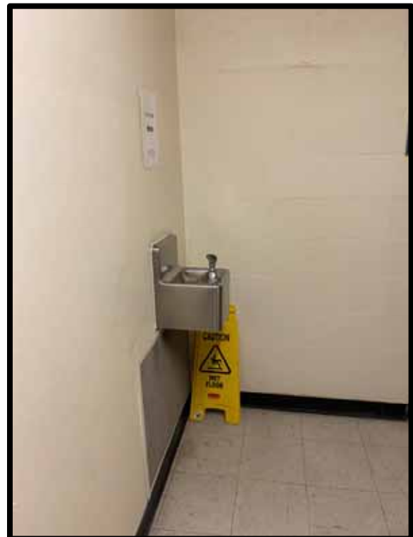
PHOTOGRAPH 230 – First floor drinking fountain. May need to be changed to meet ADA standards.
