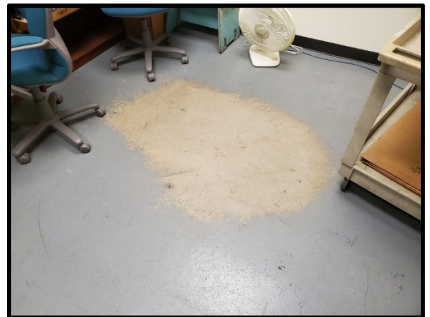
PHOTOGRAPH 72 – Example of distress to the concrete-floor staining. This type of distress is typical for buildings of this age and was only observed at isolated locations.
