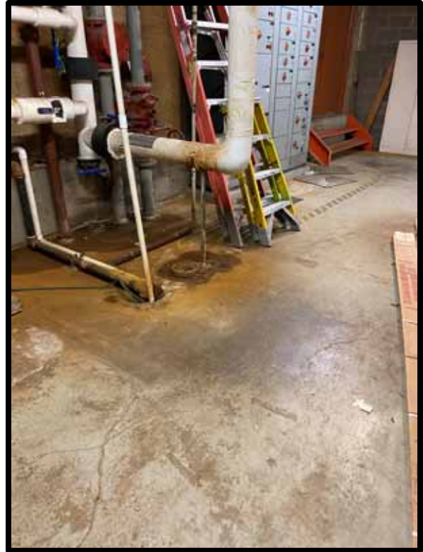
PHOTOGRAPH 265 - Mechanical room floor drain. Recommend replacement.
