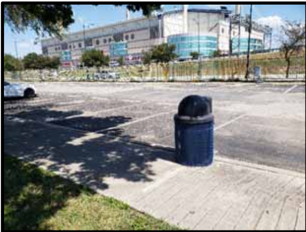
PHOTOGRAPH 3 – General view of parking lot on the east side of the property. Pavement is in fair condition with evidence of full-depth patch repairs, transverse and longitudinal cracking, raveling, and rutting.
