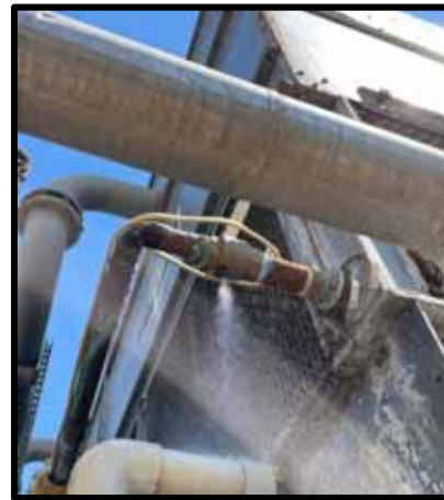
PHOTOGRAPH 108 - Cooling tower leaking valve on makeup water line
