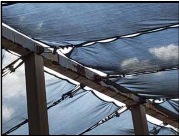
PHOTOGRAPH 39 – View of structural steel framing of the canopy structure. There is visible oxidation and possible corrosion of the steel.
