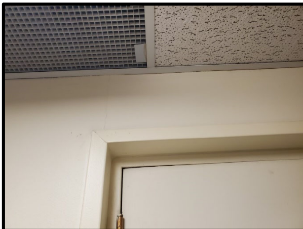
PHOTOGRAPH 77 – View of vertical crack above the door to Room 3.04.10. This type of distress is typical for buildings of this age and was only observed at isolated locations.
