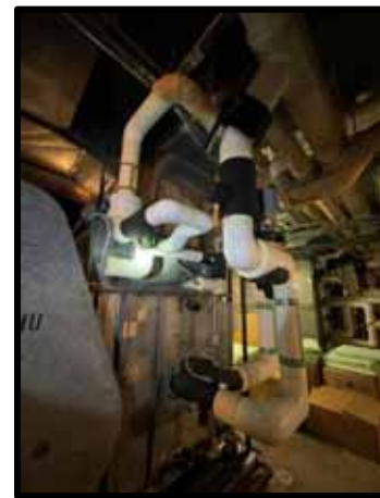
PHOTOGRAPH 138 - AHU 5 hydronic piping
