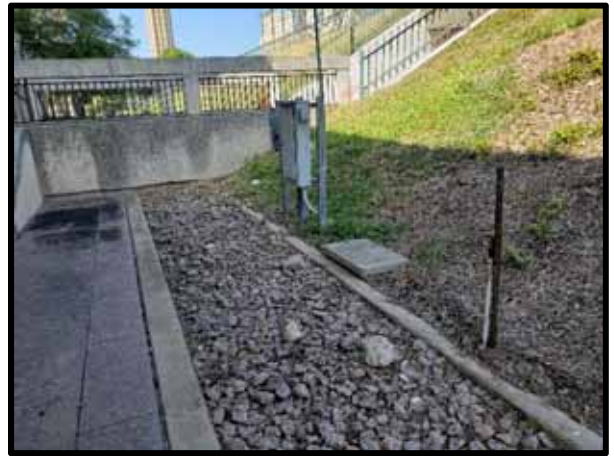
PHOTOGRAPH 32 – View of probable French drain at the base of the berm.
