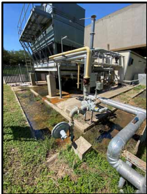
PHOTOGRAPH 311 – Gas regulator and manifold.
