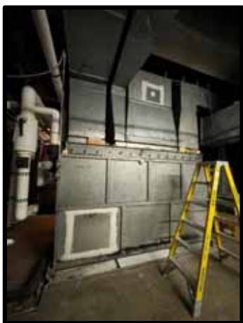
PHOTOGRAPH 131 – AHU 12 Multizone ducts
