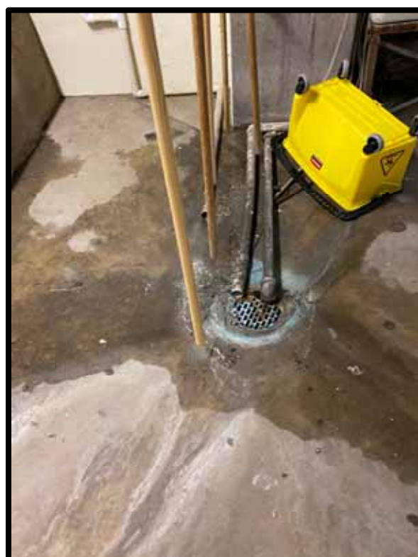
PHOTOGRAPH 262 – Mechanical room floor drain. Recommend replacement.
