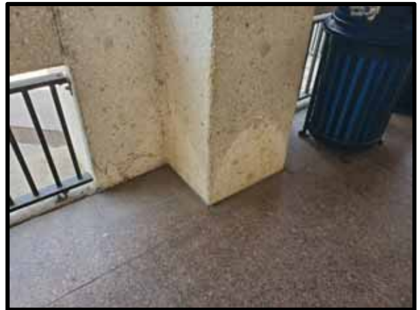
PHOTOGRAPH 46 – Example of concrete delamination at the column above the second floor balcony.
