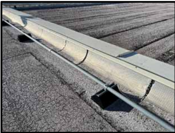
PHOTOGRAPH 57 – View of the aluminum clad base flashing and the pre-finished metal expansion joints. Aluminum clad base flashings are beginning to show signs of delamination.
