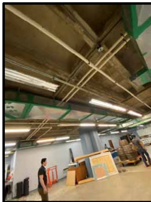
PHOTOGRAPH 299 - Storage room domestic cold and hot water piping.
