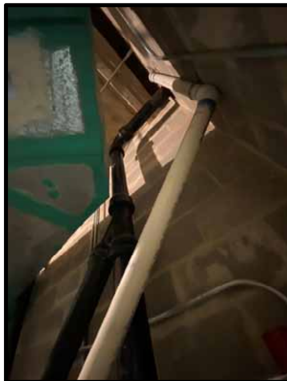
PHOTOGRAPH 258 - Sump pump piping.
