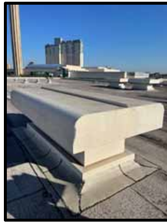
PHOTOGRAPH 168 - Outside air intake roof hoods
