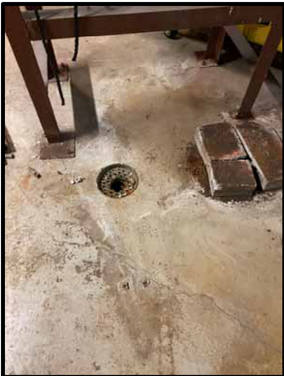
PHOTOGRAPH 264 - Mechanical room floor drain. Recommend replacement.
