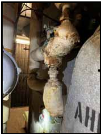
PHOTOGRAPH 115 – AHU 10 Coil piping insulation degrading
