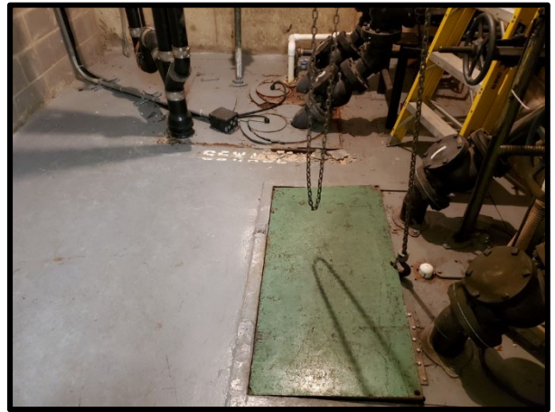
PHOTOGRAPH 74 – View of floor in Room 1.05.17. There is damage (spalls) to the concrete floor adjacent to the sump pit.
