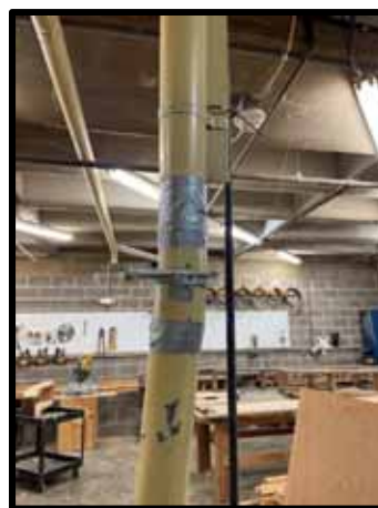
PHOTOGRAPH 188 - Damaged dust collector drop at blast gate
