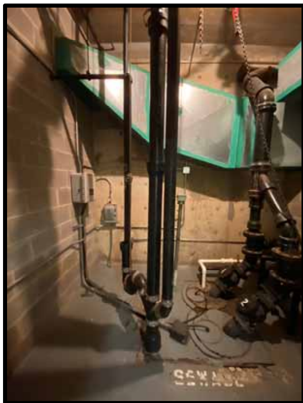
PHOTOGRAPH 259 – Cast iron piping.
