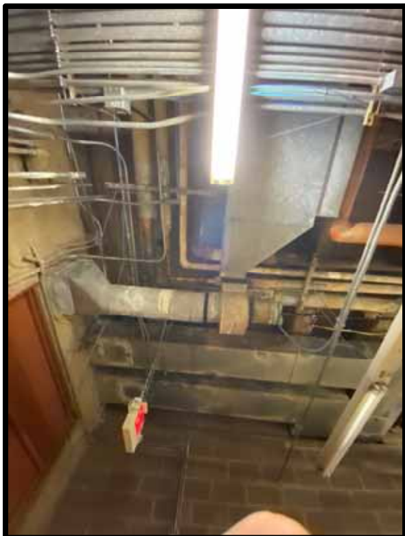
PHOTOGRAPH 288 – Typical domestic cold and hot water piping. Missing insulation
