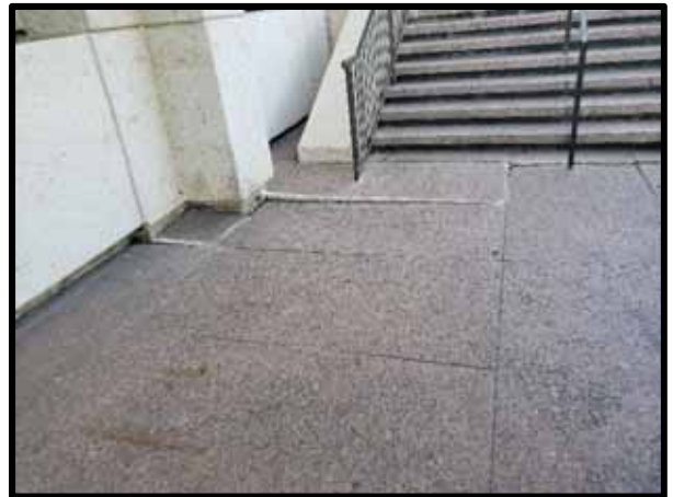
PHOTOGRAPH 22 – View of granite sidewalk with possible settlement of the sidewalk adjacent to the building foundation and stairs. The differential movement of the granite sidewalk has created a trip hazard which is a life-safety issue.
