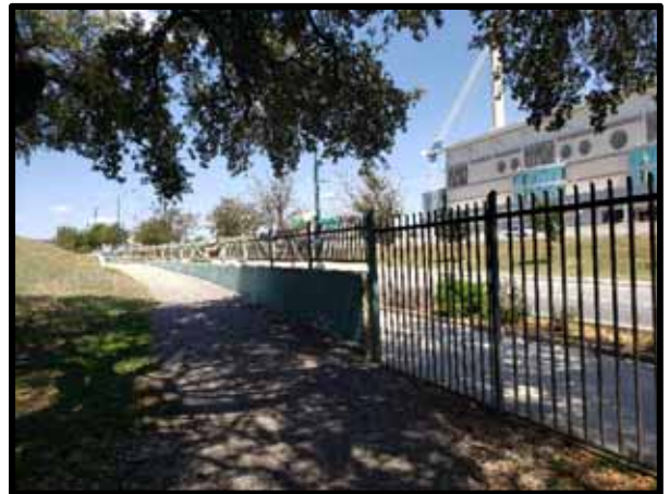
PHOTOGRAPH 28 – General view of fencing along east property boundary. Fencing has chipped and peeling paint, surface oxidation, and possible corrosion.
