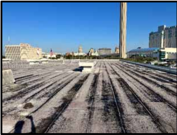
PHOTOGRAPH 55 – View of existing modified bitumen roofing system. Granule loss and membrane alligatoring is typical in the roofing membrane.
