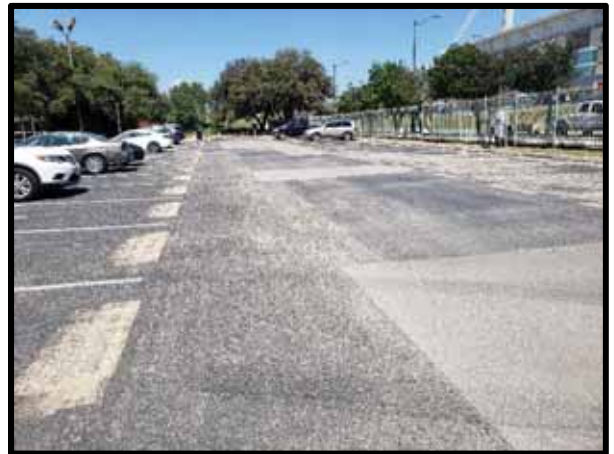
PHOTOGRAPH 4 - General view of parking lot on the east side of the property. Pavement is in fair condition with evidence of full-depth patch repairs, transverse and longitudinal cracking, raveling, and rutting.
