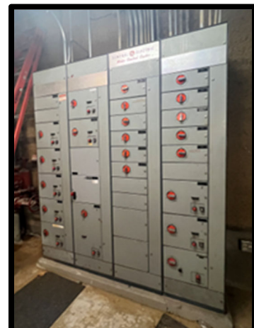
PHOTOGRAPH 192 – Motor Control Center example
