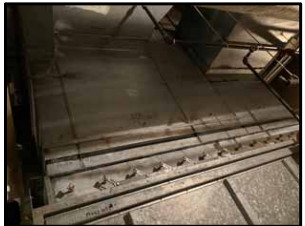
PHOTOGRAPH 164 - AHU 13 Damper system
