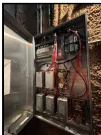
PHOTOGRAPH 158 - AHU 8 Controls
