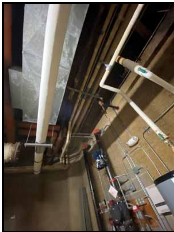
PHOTOGRAPH 282 - Typical domestic cold and hot water piping.
