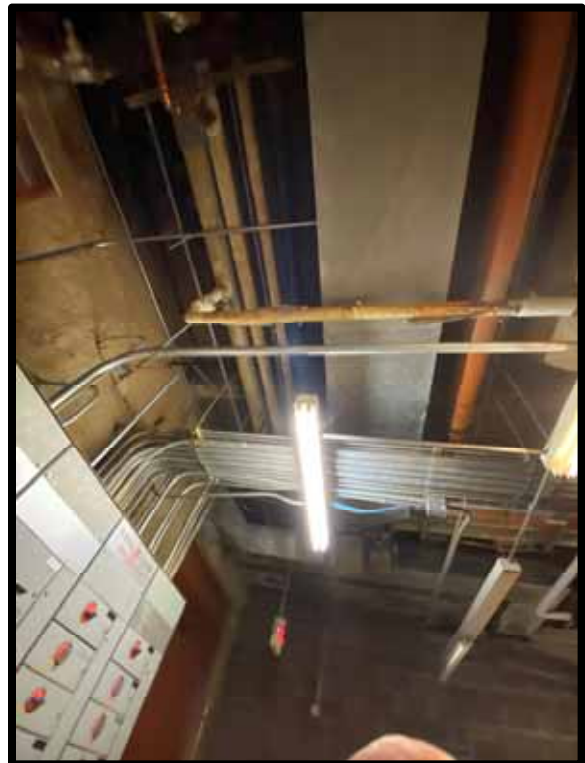
PHOTOGRAPH 287 – Typical domestic cold and hot water piping. Damaged insulation.
