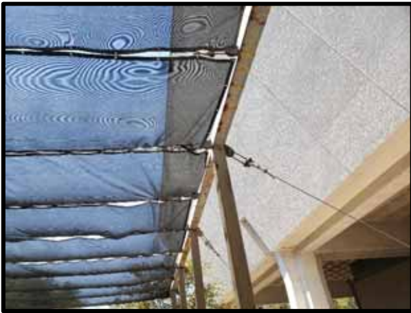
PHOTOGRAPH 37 – View of structural steel framing of the canopy structure. There is visible oxidation and possible corrosion of the steel.
