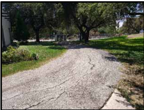
PHOTOGRAPH 17 – View of asphalt sidewalk that extends along the east side of the property. Pavement is in poor condition with transverse and longitudinal cracks and edge raveling.
