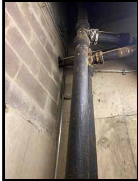
PHOTOGRAPH 249 – Possible leak from cast iron.
