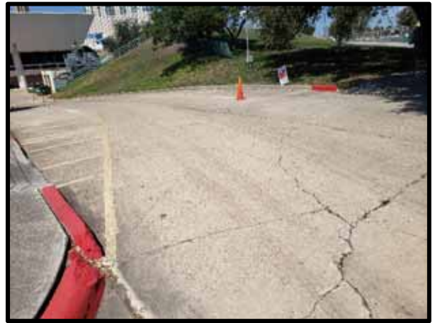
PHOTOGRAPH 8 - View of the service drive with transverse and longitudinal cracks.
