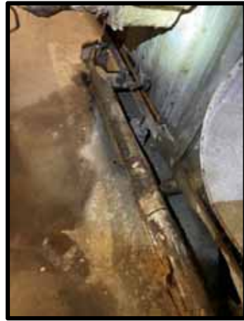
PHOTOGRAPH 114 - AHU 10 Condensate Piping insulation degradation
