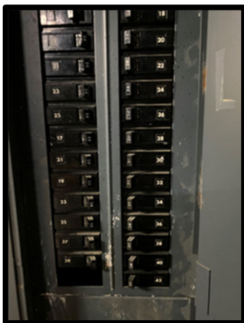
PHOTOGRAPH 195 – Example of Panel missing blank cover
