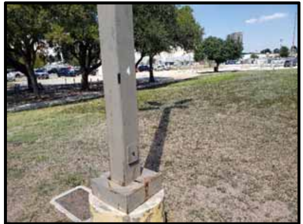
PHOTOGRAPH 34 – View of light pole with surface oxidation and possible corrosion around the base of the pole.
