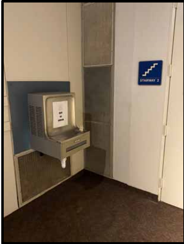
PHOTOGRAPH 231 – Second floor drinking fountain. May need to be changed to meet ADA standards.
