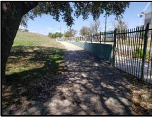
PHOTOGRAPH 19 – View of asphalt sidewalk that extends along the east side of the property. Pavement is in poor condition with transverse and longitudinal cracks and edge raveling.
