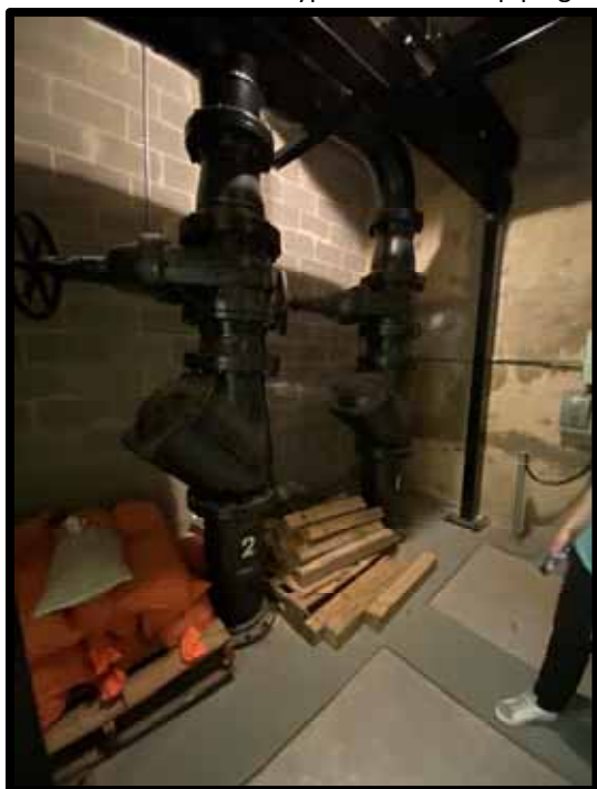
PHOTOGRAPH 274 – Roof drain sump pump piping.
