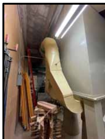
PHOTOGRAPH 184 – Duct at rear of Dust collector unit
