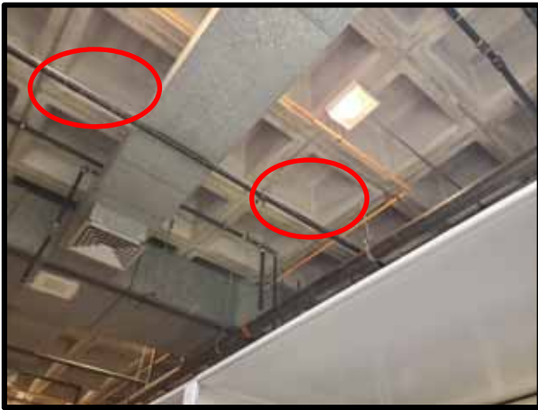
PHOTOGRAPH 49 – View of roof framing with possible moisture staining.
