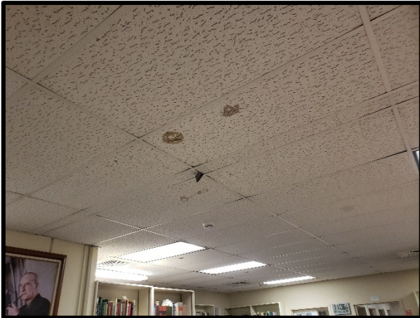
PHOTOGRAPH 81 – Example of staining on the ceiling tiles.
