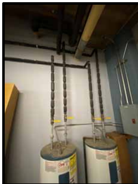
PHOTOGRAPH 294 – Storage room water heaters. CW line needs heat trap, vacuum breaker, and expansion tank.
