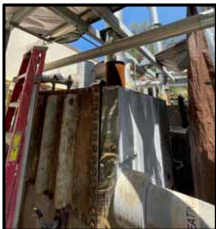
PHOTOGRAPH 103 – Corrosion on back side of Boiler 1
