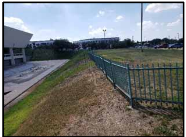
PHOTOGRAPH 30 – View of fencing on top of the berm to the west of the building. The fence is leaning and several of the footings appear to be undermined. Shoring has been installed to prevent collapse of the fence.
