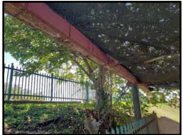
PHOTOGRAPH 40 – View of structural steel framing of the canopy structure. There is visible oxidation and possible corrosion of the steel.
