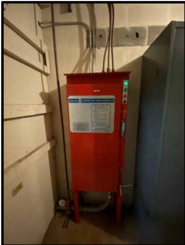
PHOTOGRAPH 318 – Fire pump controller.
