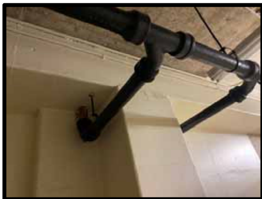
PHOTOGRAPH 236 – Typical cast iron piping.
