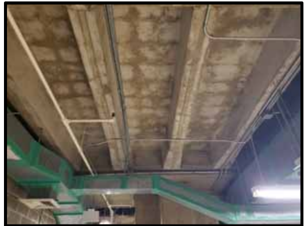
PHOTOGRAPH 52 - View of second floor framing with staining that may indicate moisture infiltration.
