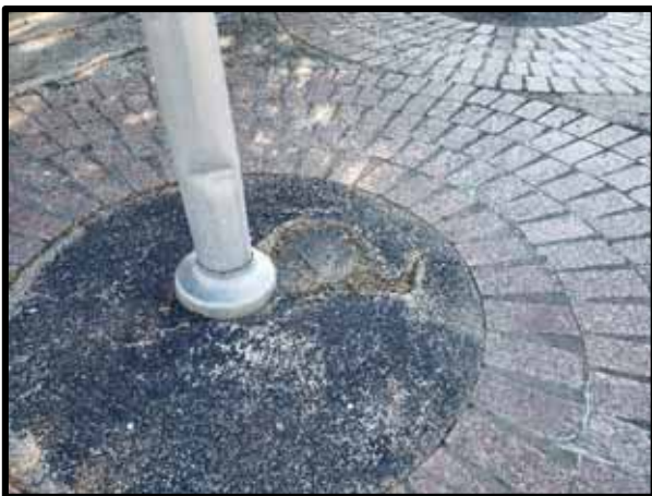
PHOTOGRAPH 41 – Example of dented flagpole.
