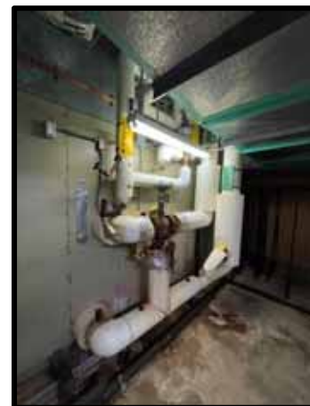
PHOTOGRAPH 124 – AHU 17 Corroded hydronic piping and damaged insulation
