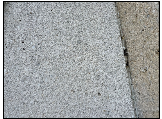
PHOTOGRAPH 70 - Sealant joint failure at the fountain and walkover bridge area.
