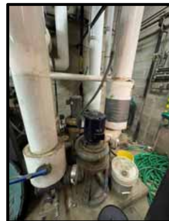
PHOTOGRAPH 94 – Piping to hot water pumps
