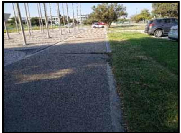
PHOTOGRAPH 10 – View of concrete sidewalk on the west side of the property. The sidewalk has evidence of differential movement and is considered a trip hazard. Trip hazards are a life safety issue.
