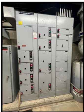
PHOTOGRAPH 193 – Motor Control Center example
