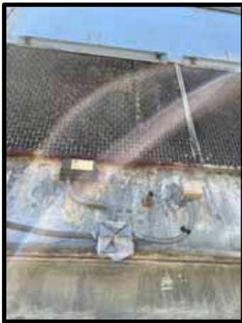
PHOTOGRAPH 107 – Cooling tower corrosion and wear
