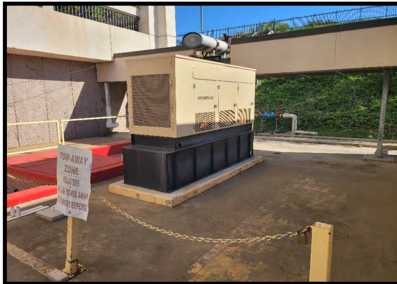
Photo 19. Natural gas generator on SITE.
