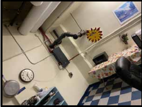
PHOTOGRAPH 247 – Typical cast iron piping. Verify that cast iron is a minimum of 6' from floor.
