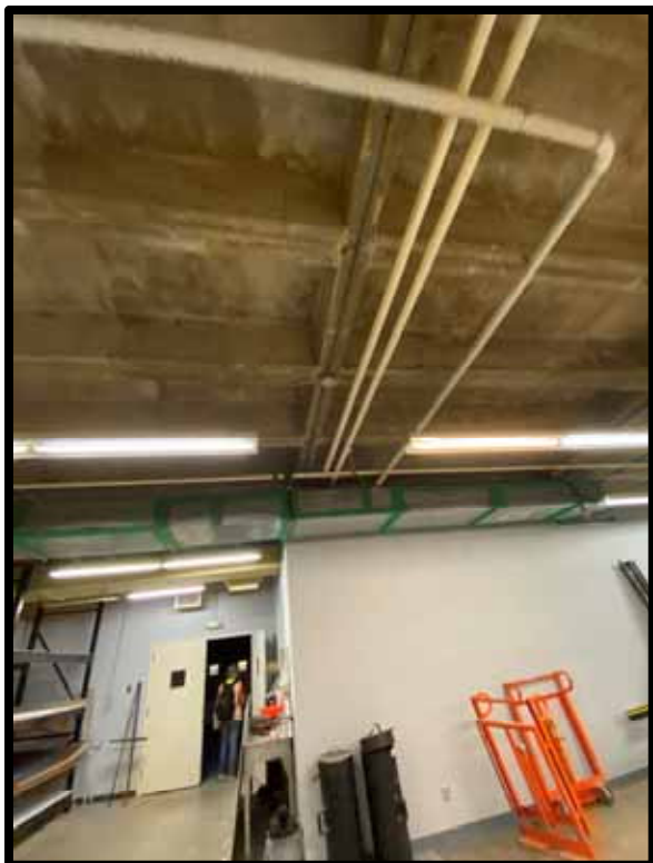
PHOTOGRAPH 300 - Storage room domestic cold and hot water piping.
