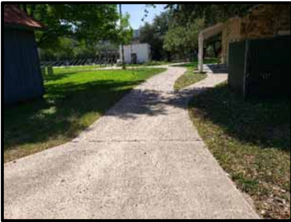
PHOTOGRAPH 13 – General view of the concrete sidewalk with exposed aggregate and aggregate pops.
