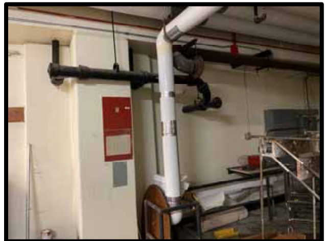
PHOTOGRAPH 246 - Typical cast iron piping.
