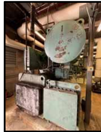
PHOTOGRAPH 84 - Chiller 1 Evaporator insulation degrading
