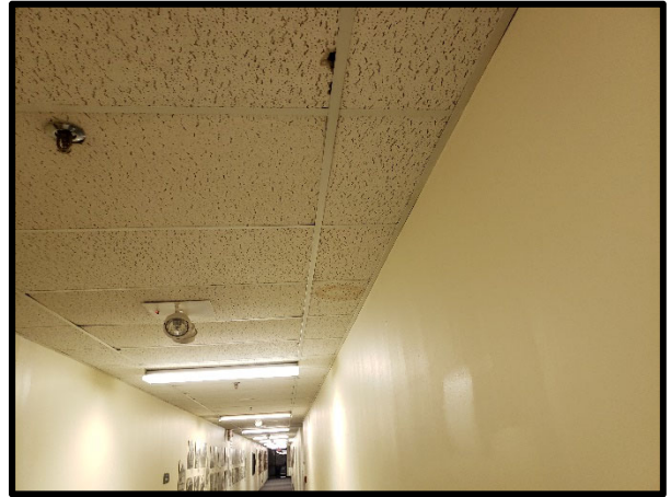
PHOTOGRAPH 80 – General view of ceiling tiles in Corridor 3.04.C4. Typical distress conditions include staining and broken or damaged tiles. This type of distress is typical for buildings of this age and was only observed at isolated locations.
