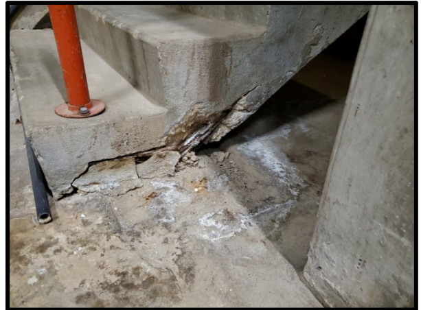
PHOTOGRAPH 82 – View of interior stairs with spalled concrete and exposed rebar. The rebar has severe corrosion with significant loss of section. This is located in the mechanical pit with the chiller units.
