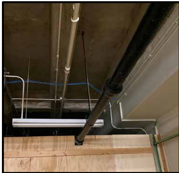
PHOTOGRAPH 237 - Typical cast iron piping.
