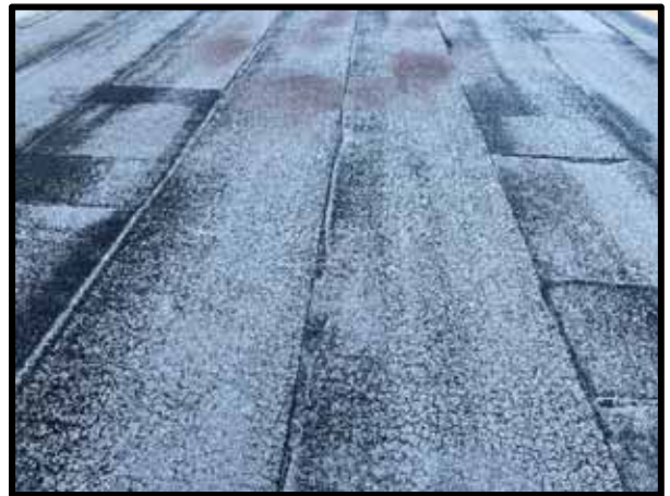
PHOTOGRAPH 58 – View of membrane alligatoring and membrane shrinkage in the modified bitumen roof membrane.
