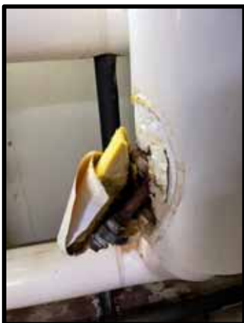
PHOTOGRAPH 123 – AHU 17 Corroded strainer on chill water supply, damaged insulation
