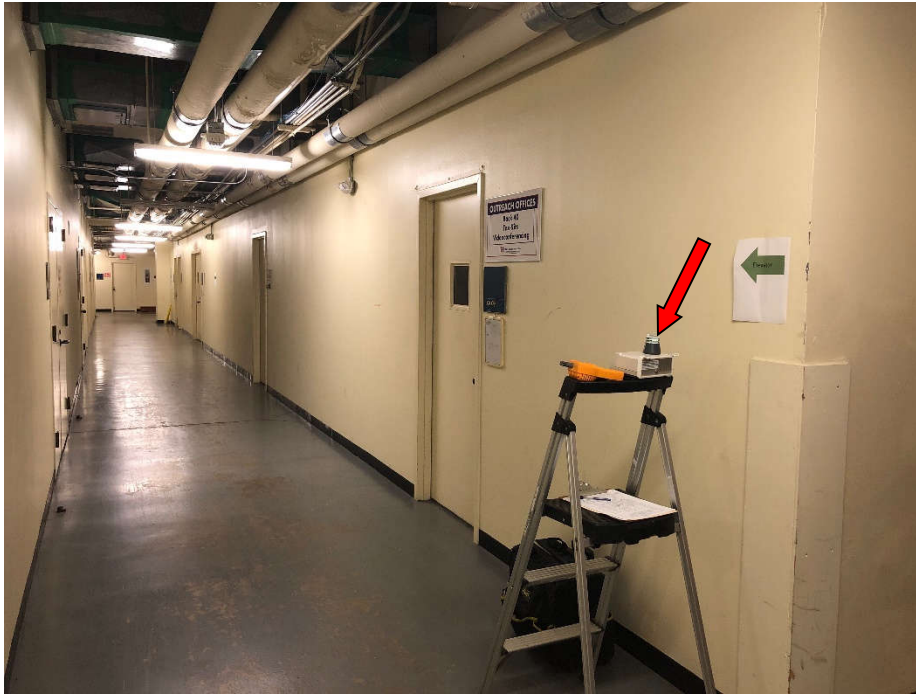
PHOTO 5: Shows airborne mold sample BZ-05, indicated by the red arrow, collected from the normal breathing zone in Corridor 1.04 by Restroom 1.04.09.
