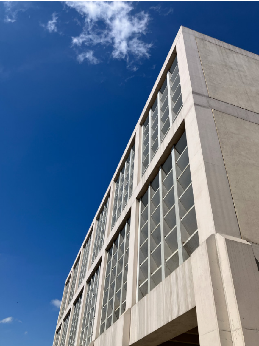
STEP - Cooling Towers
