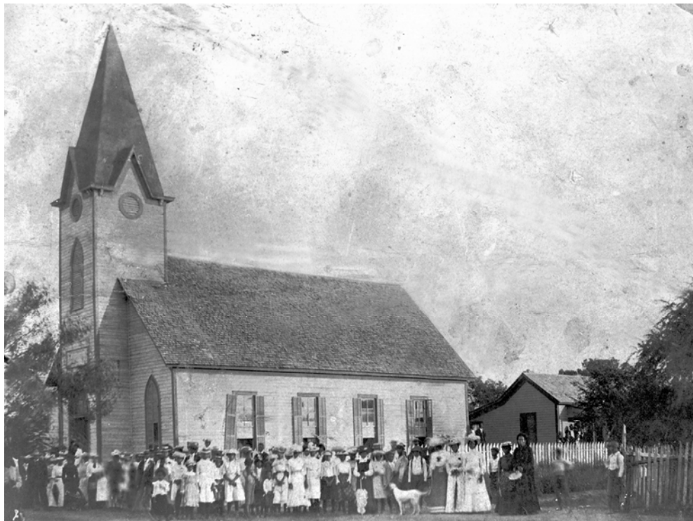
Mount Zion First Baptist Church's original location on Santos Street in the Baptist Settlement. Source: UTSA Special Collections.
