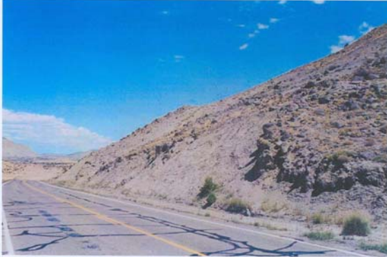
Figure 4. This picture is showing a relatively smooth slope with low level launching features. This would have a RHRS rating of 3 points.
